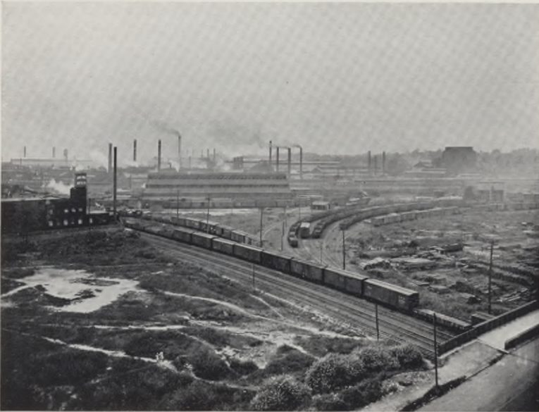
DIE ANLAGE DER MIDVALE STEEL COMPANY, WAYNE JUNCTION, PHILADELPHIA
