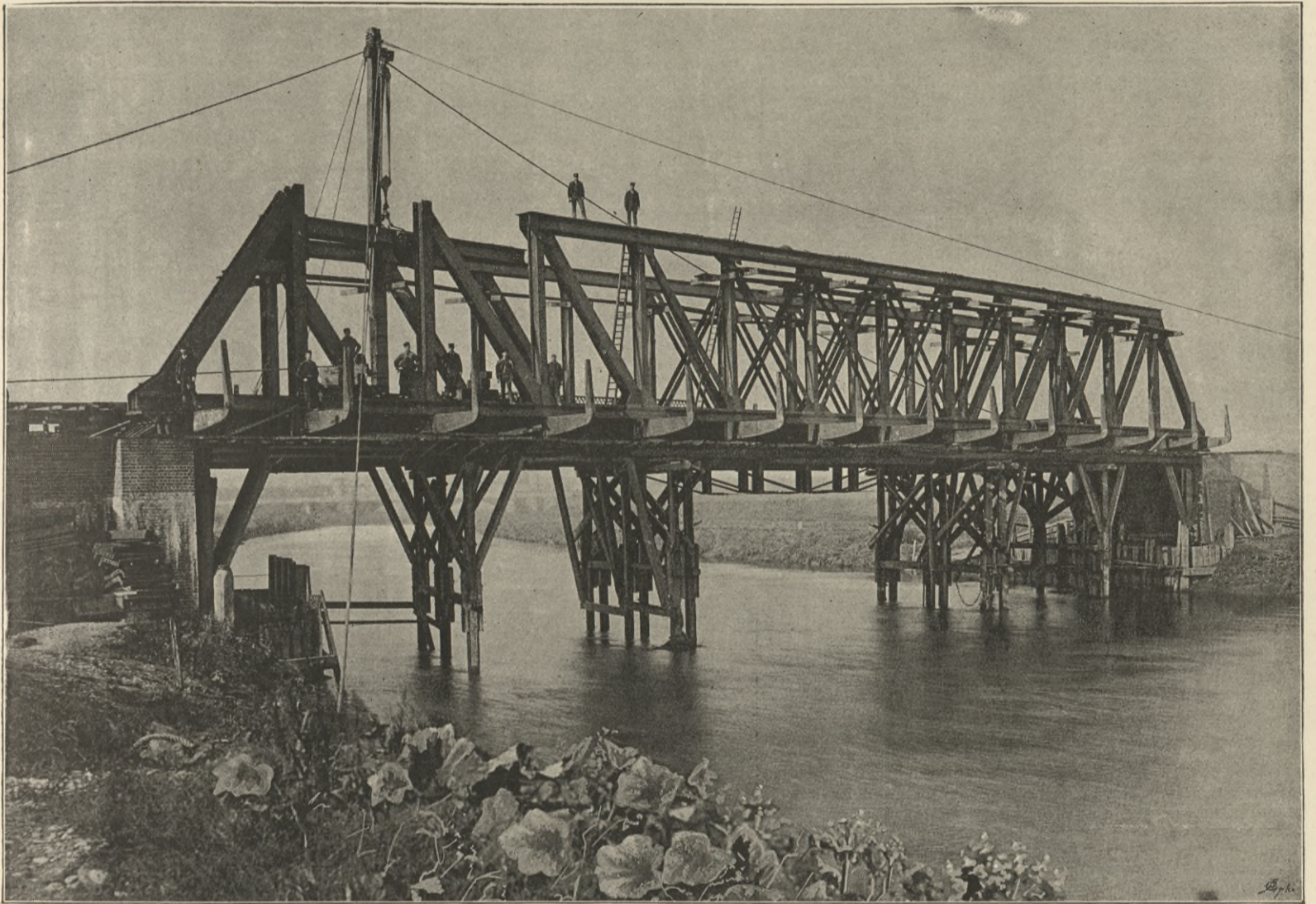
FIG. 24. BRIDGE OVER RIVER MERSEY; RAILWAY DEVIATION No. 1. (See Page 18.)
