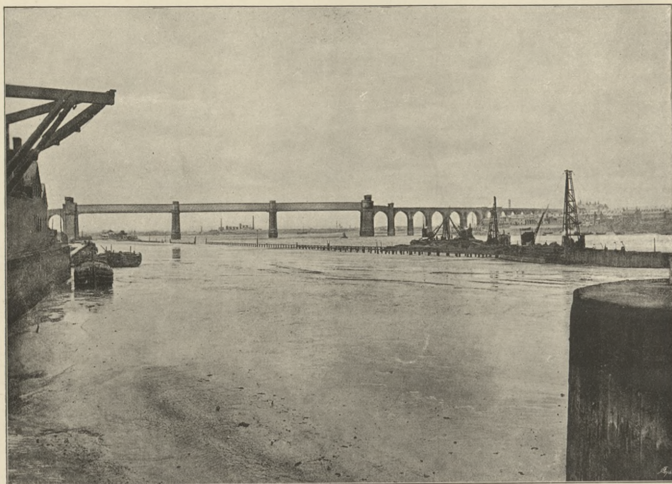
FIG. 10. RUNCORN VIADUCT; LONDON AND NORTH-WESTERN RAILWAY.
