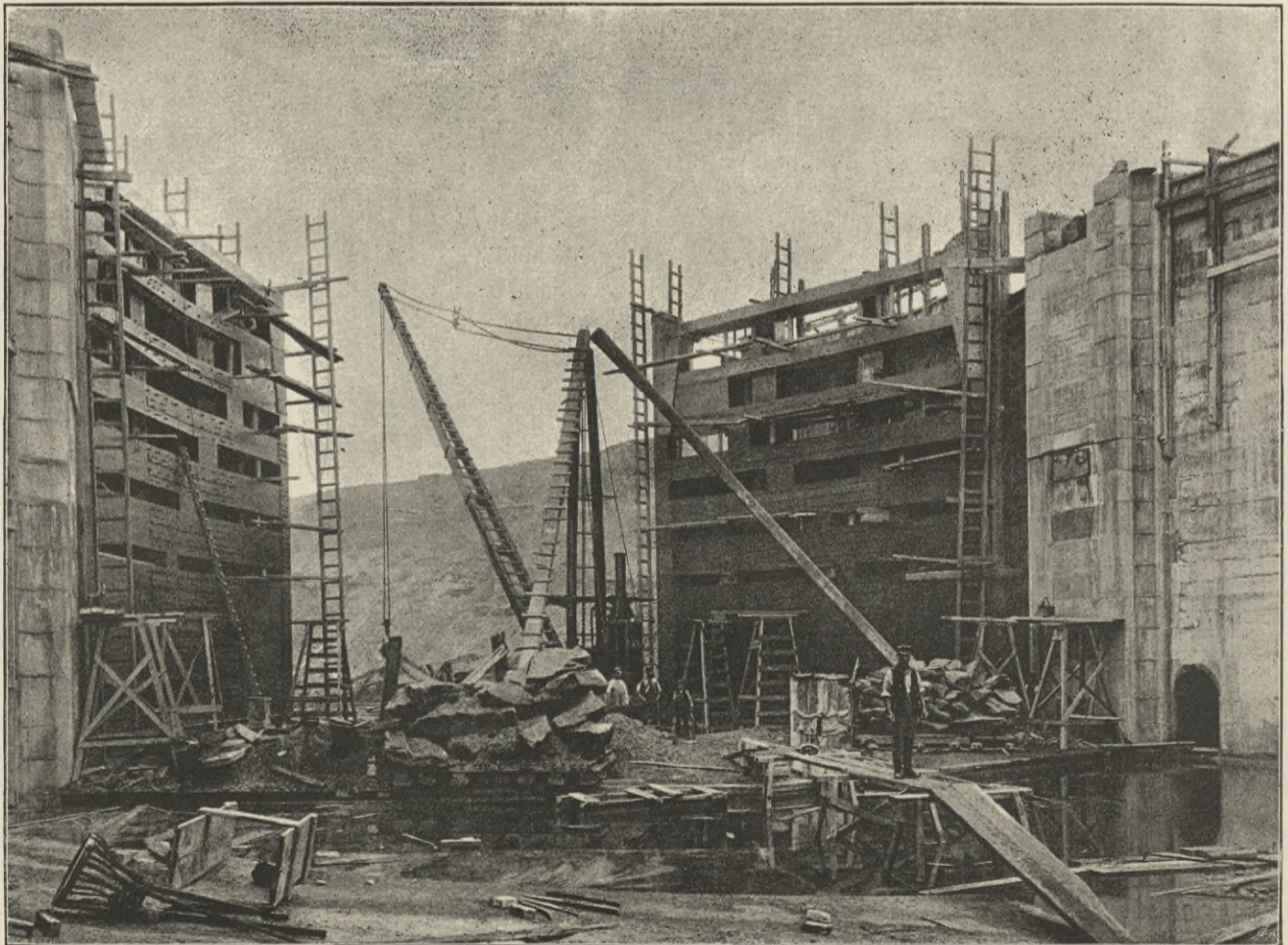
FIG. 4. 80-FT. GATES, EASTHAM LOCK. (See Page 14.)
