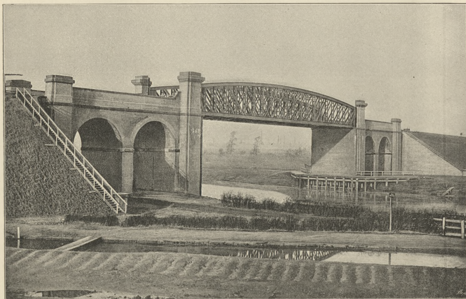
FIG. 11. BRIDGE OVER THE RIVER MERSEY; RAILWAY DEVIATION NO 1.
