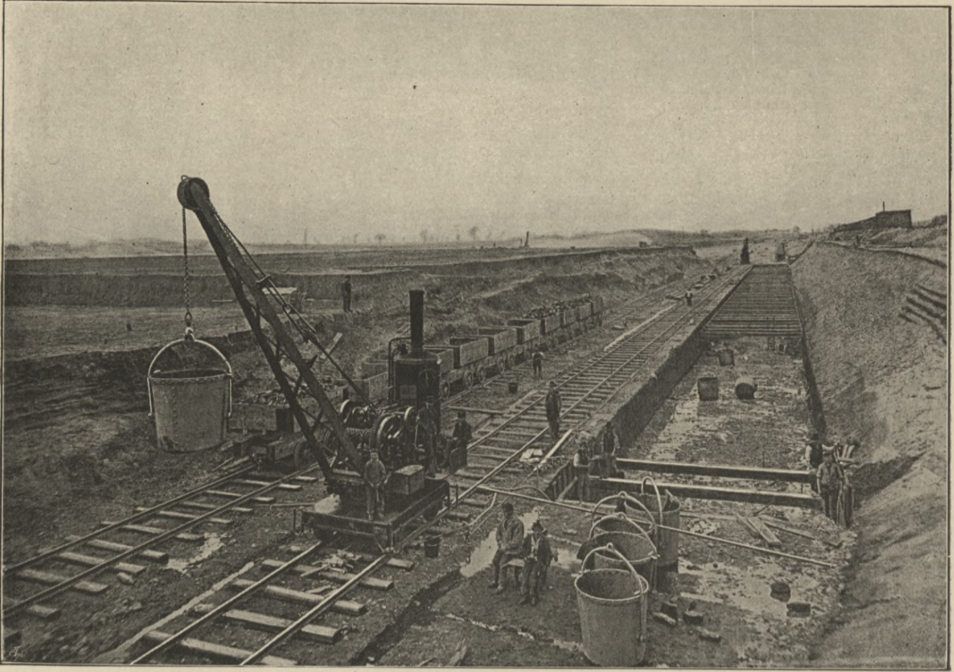
FIG. 158. LAYING FOUNDATIONS OF QUAY WALLS FOR SALFORD DOCKS. (See Page 35.)
