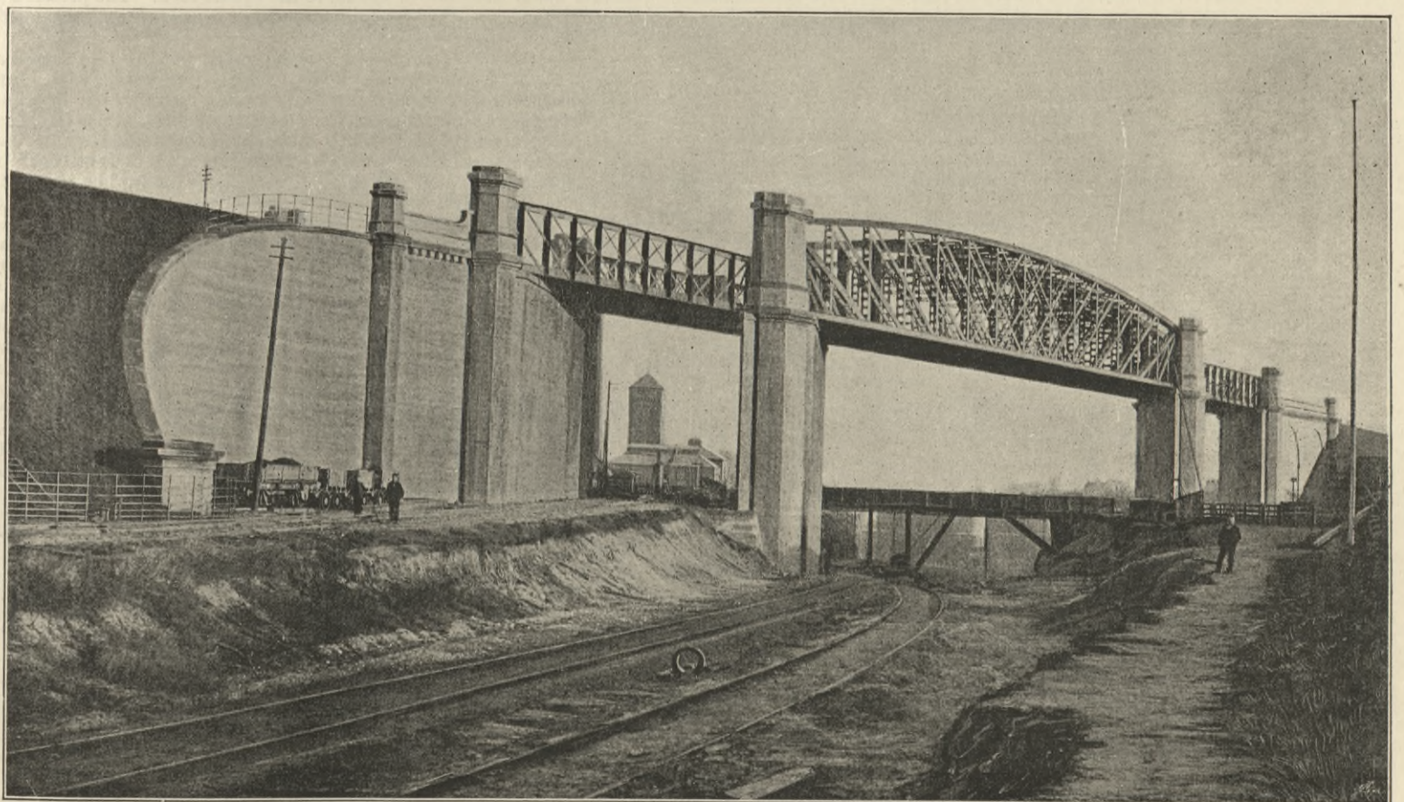
Fig. 25. BRIDGE OVER CANAL; RAILWAY DEVIATION No. 3. (See Page 19.)
