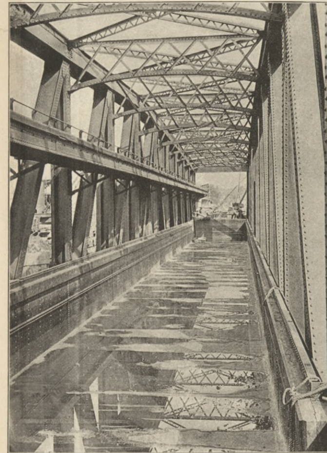
FIG. 85. INTERIOR OF THE AQUEDUCT.
