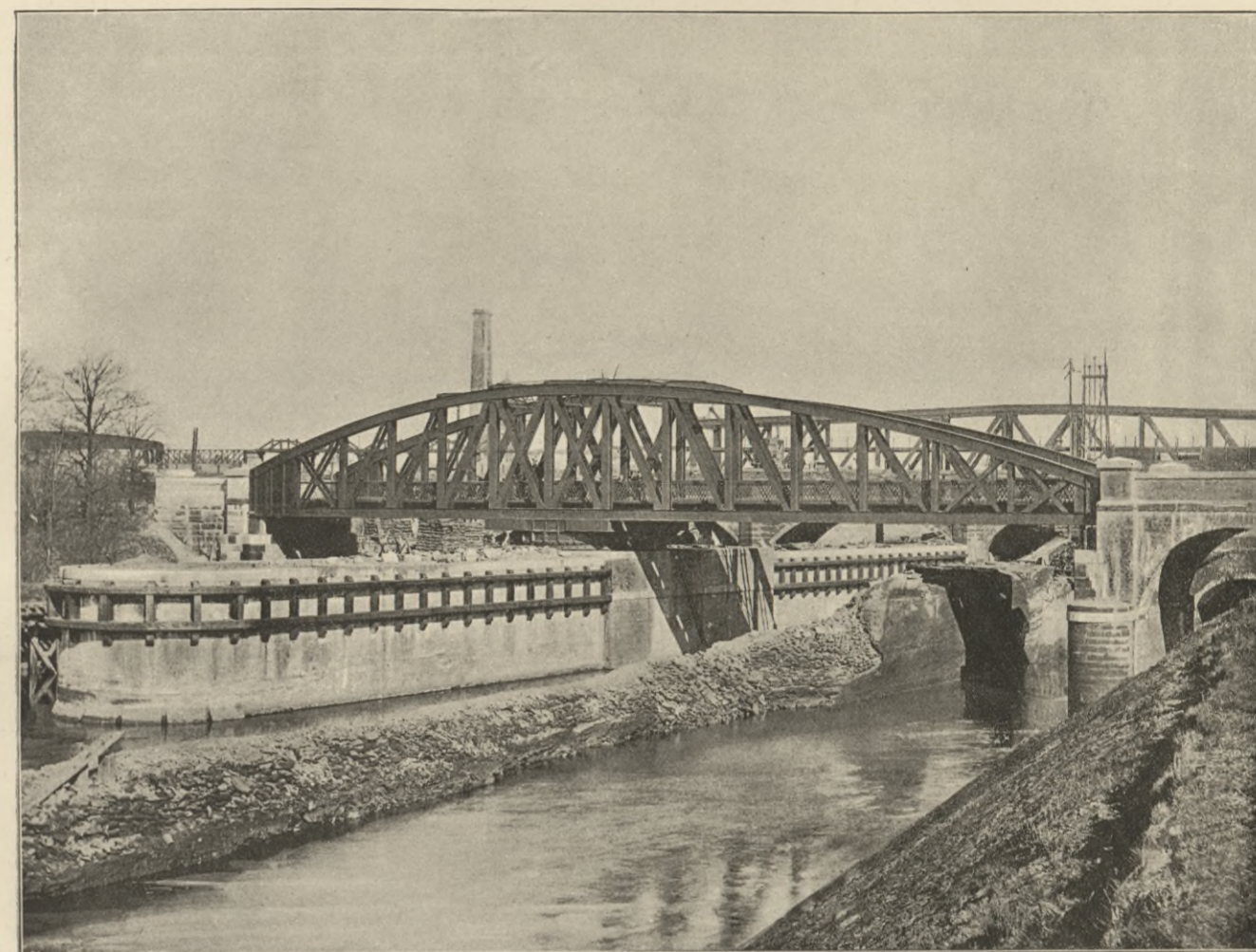
FIG. 12. BARTON SWING BRIDGE.
