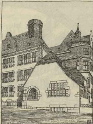
Gymnasium Zeilendoor, Arch. Theodor Frankfurter
