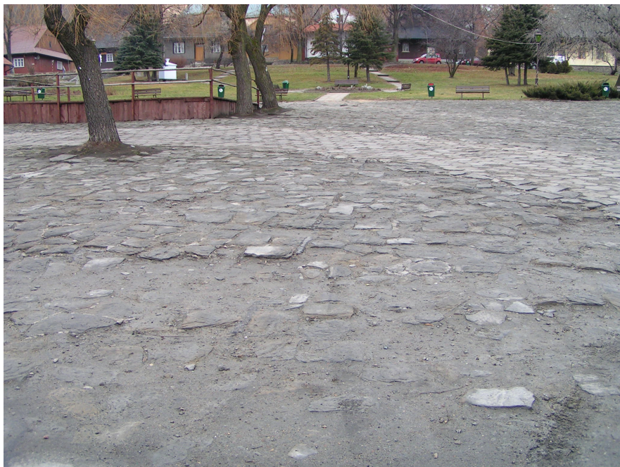
Fig. 5. Condition of the surface of the market square prior to the renovation: 1 – lower part; 2. upper part, 2003 (by A. Mitkowska)
