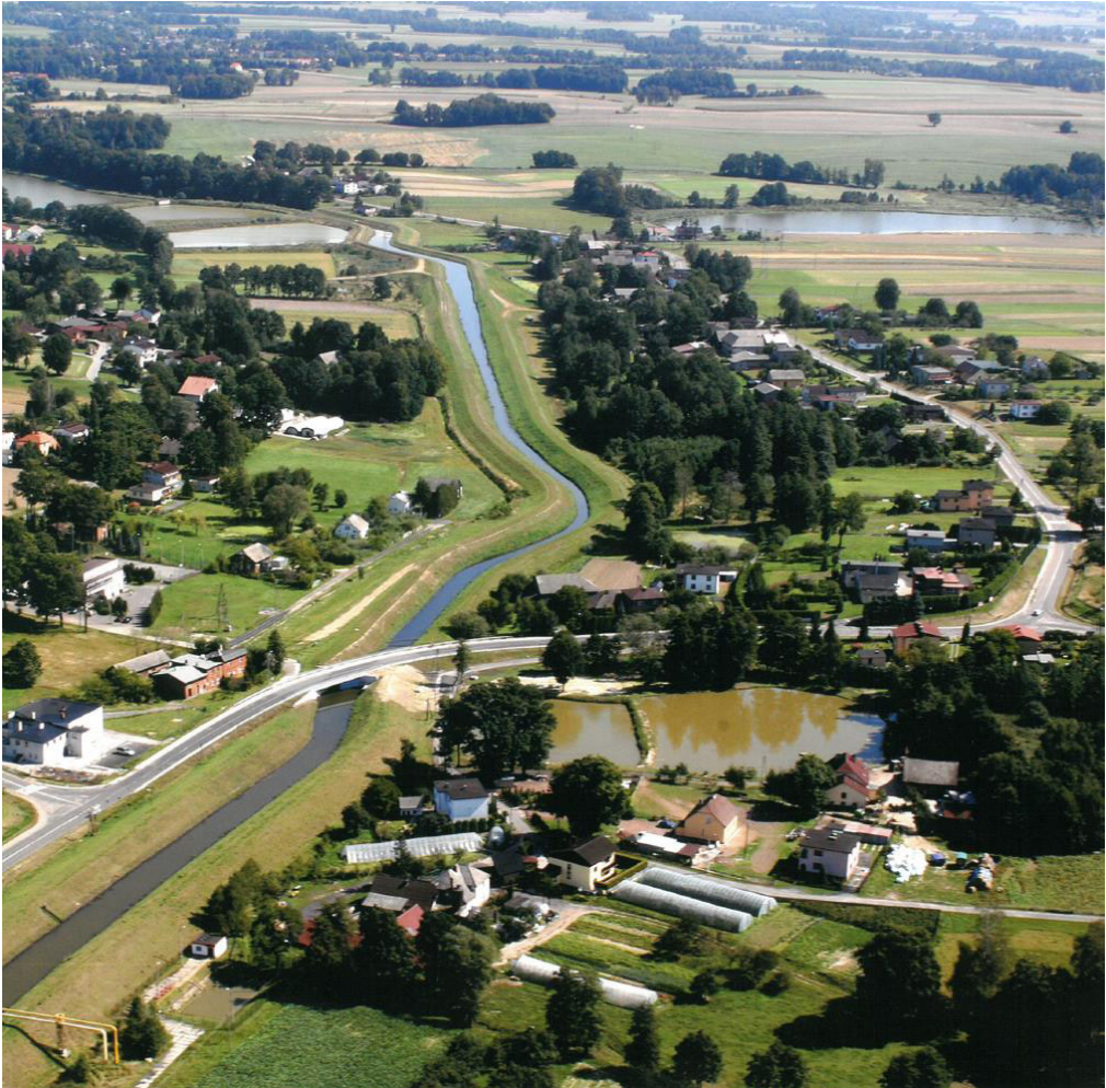
Fig. 10. Completed works after the most recent restoration
