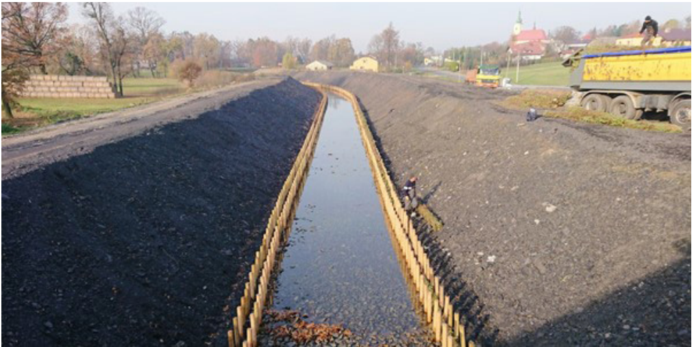
Fig. 9. Fascine construction works
