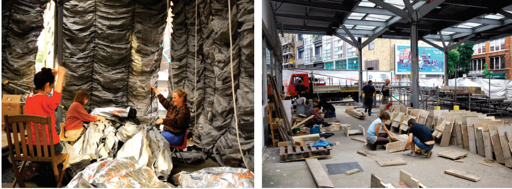
Fig. 3. Assemble, The Cineroleum (work in progress) photo by Assemble [7]
