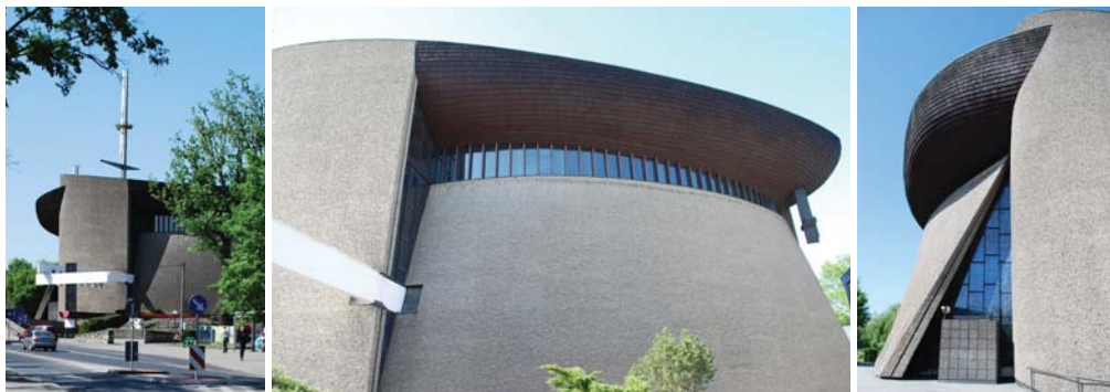
Fig. 1–3. The Ark of the Lord Church visible from the south (source: author's own archives)
