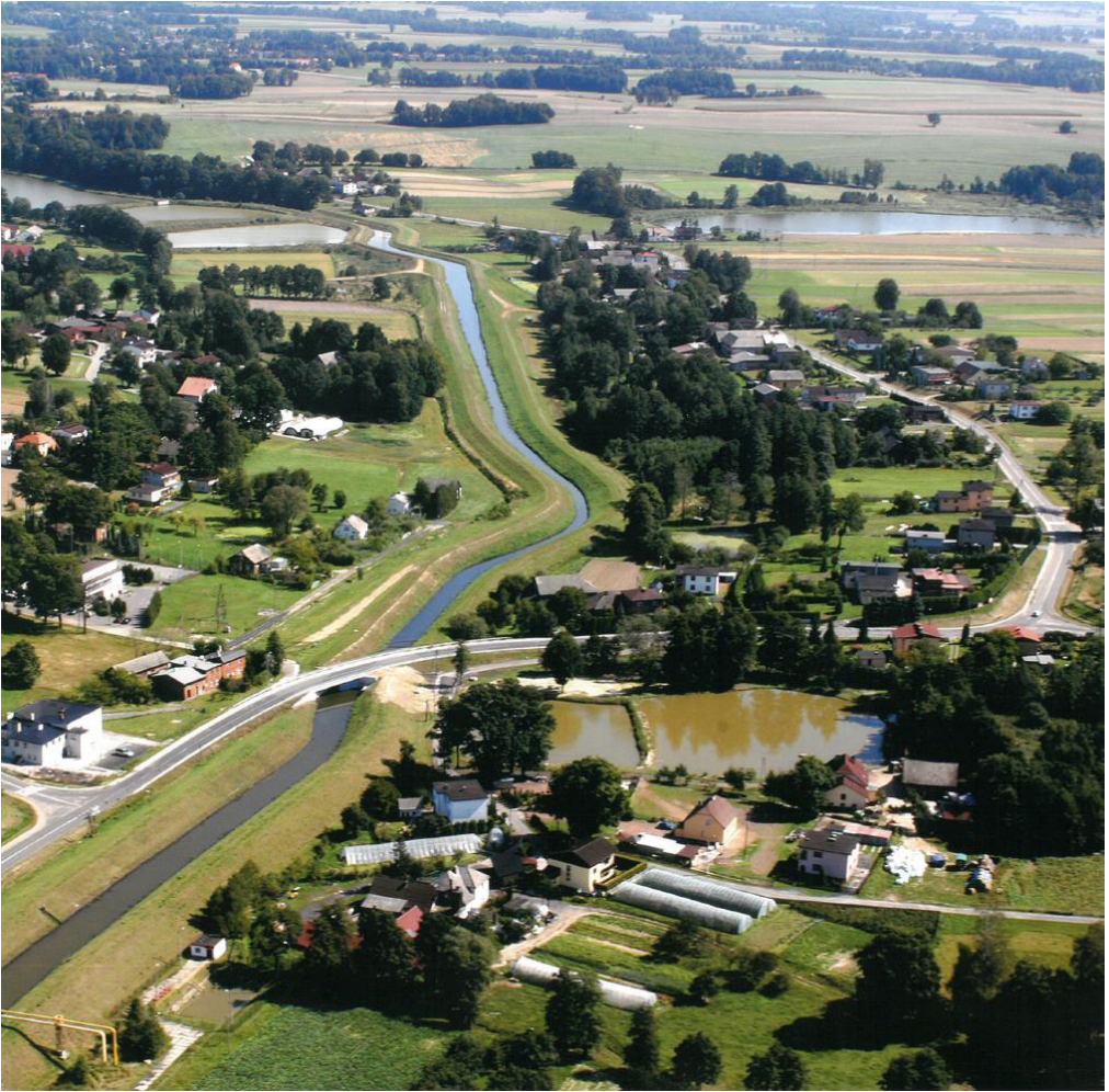
Fig. 10. Completed works after the most recent restoration
