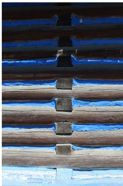
Figure 8 - Detail of blue painted gaps between wooden framework beams and blue primed plinth in Tylmanowa village (photo by Justyna Tarajko-Kowalska 2015)
