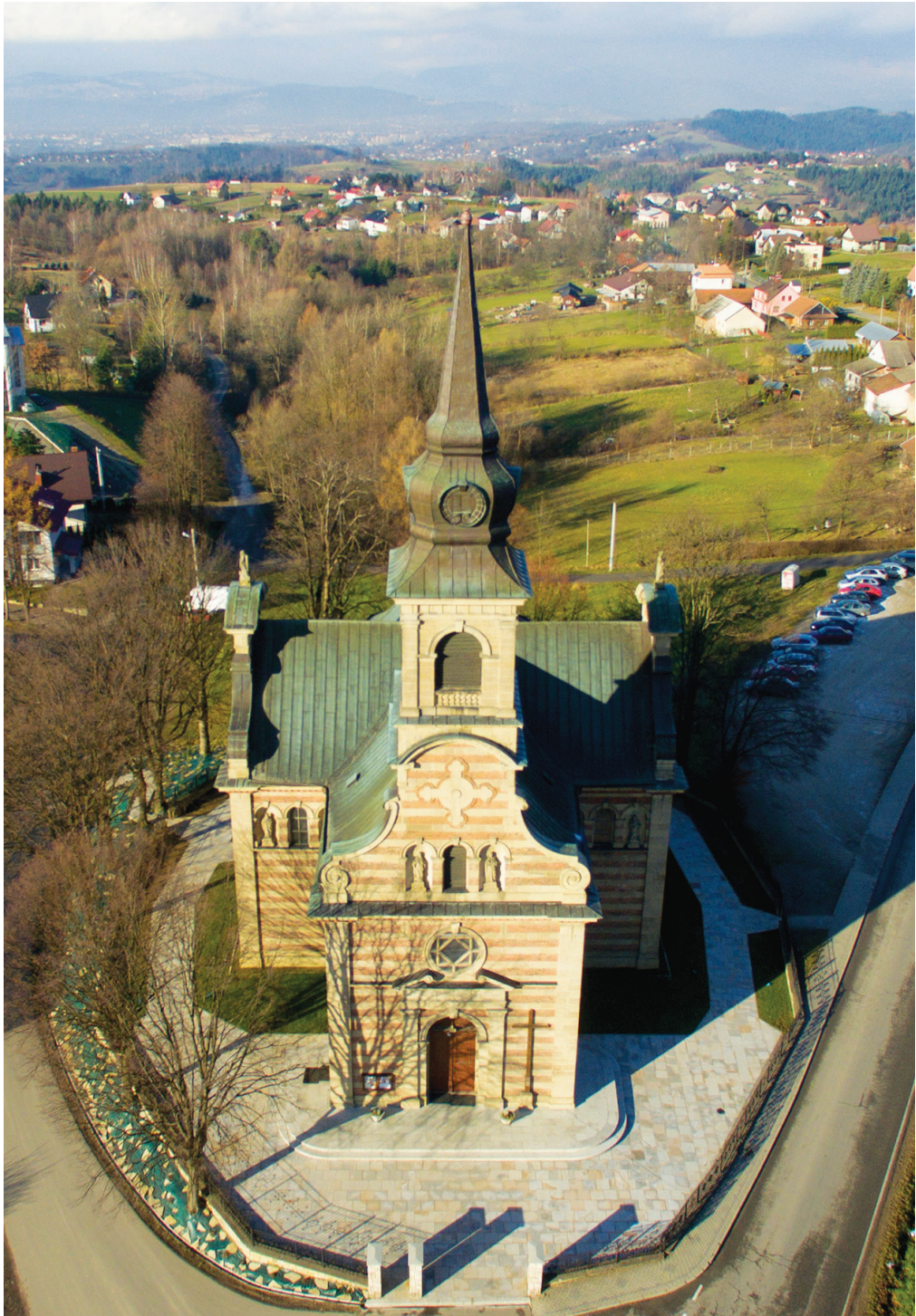
Fig. 4. Parish church in Mystkow – main entrance façade, photo by Kamil Ogórek
