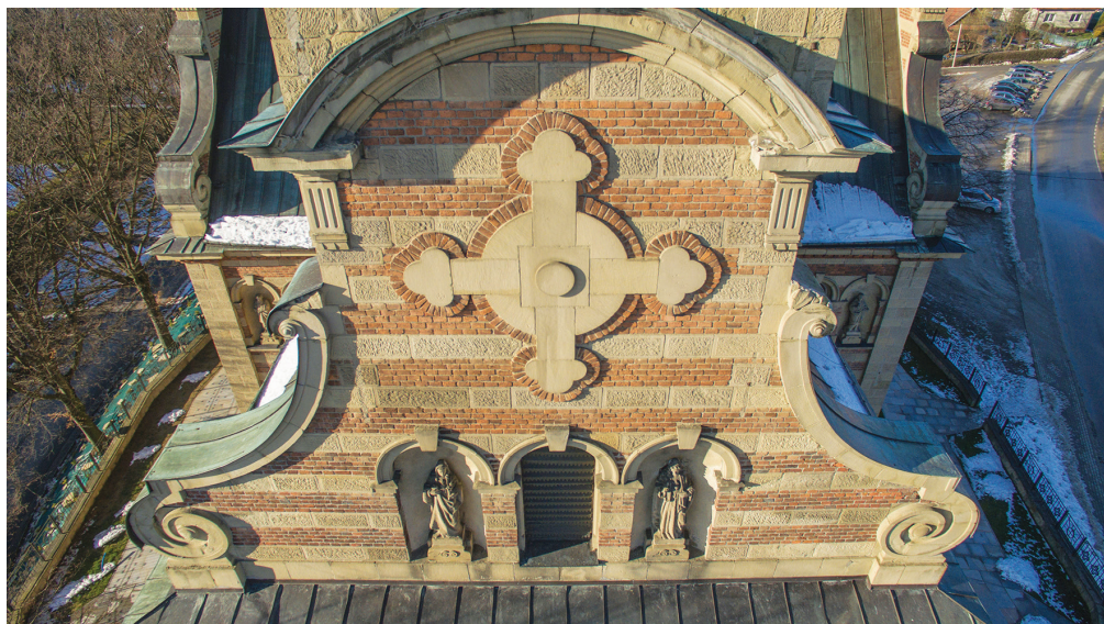
Fig. 2. Parish church in Mystków – façade details
