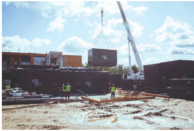
III. 2. Modular Hotel Extension: Bonifacio Spa and Sport Resort, Sochocin, n/Warsaw, Poland. View of the assembling phase. The turn key guestrooms are connected on site. Photo: DMDmodular
