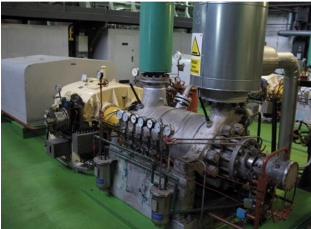
Fig. 1. Steam water pump for the Z-type steam boiler
