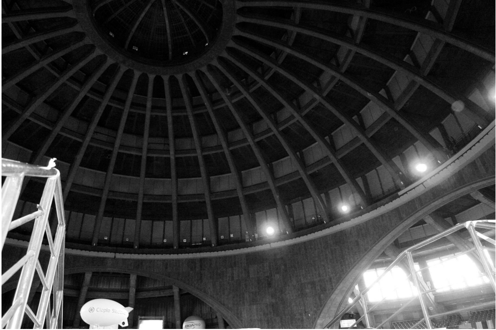
III. 2. Hala Stulecia in Wrocław, Max Berg, phot. T.B-B
