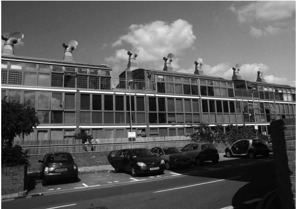
III. 5. The BedZED housing development, the form exhibits the eco-friendly solutions in place at the estate, phot. A. Bonenberg
