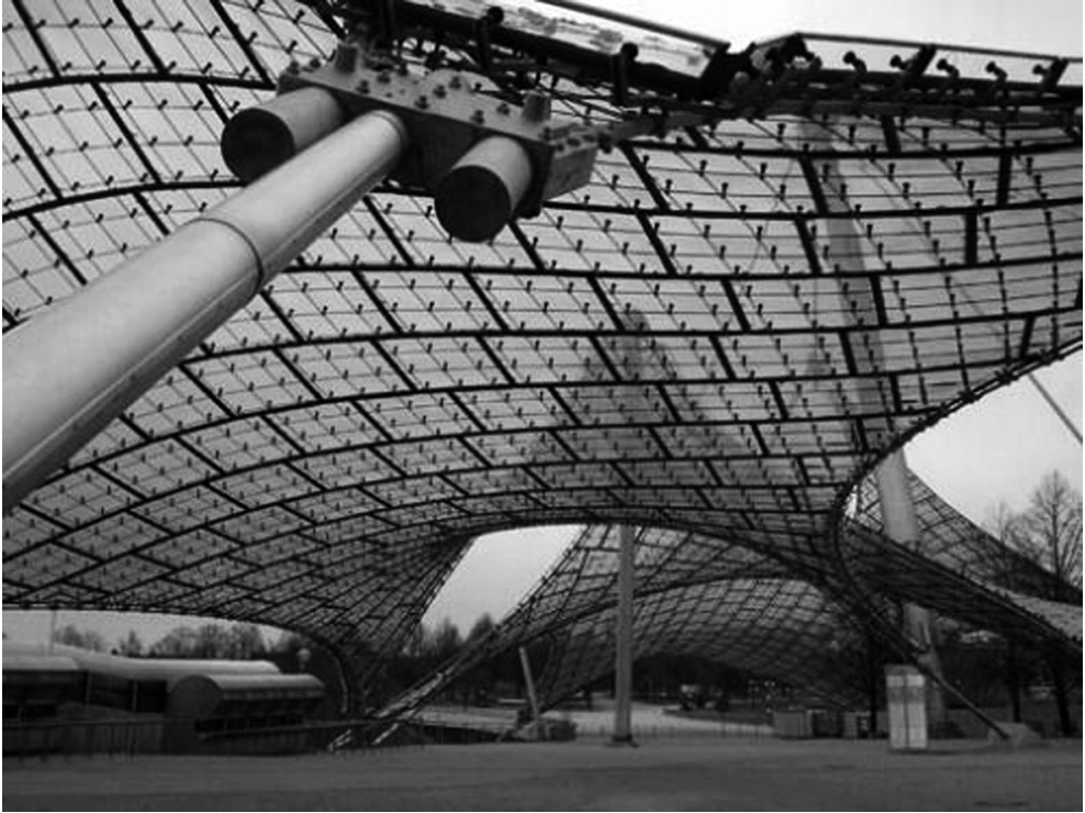
III. 3. Roofing of the Olympic complex in Munich, phot. E. Tarka
