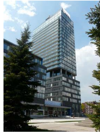
Figure 24. Regent Park's 22- story building with district heating plant. Source: D. Pollard
