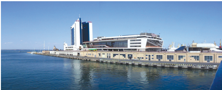
III. 4. View of the terminal in 2001–2015
