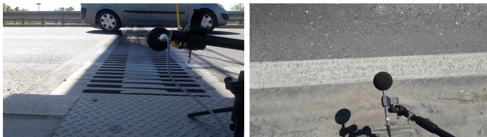
Fig. 3. a) Microphone location above the dilatation b) Microphone location at the base point
