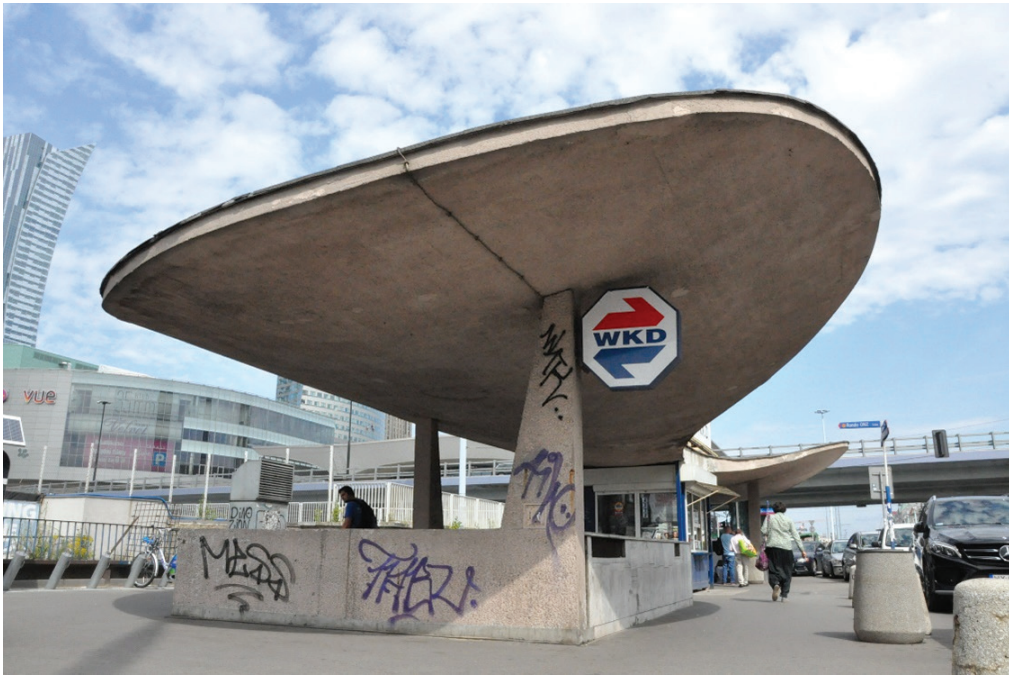
Fig. 2. Reinforced concrete canopy at the Warsaw Śródmieście WKD railway station [by author]
