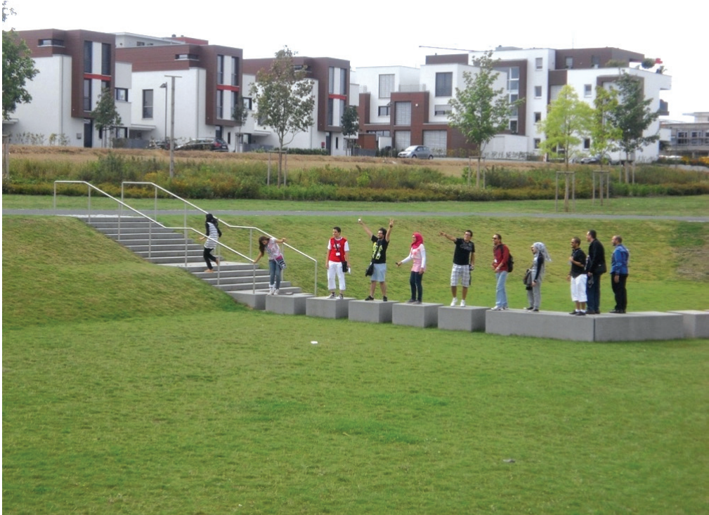
Fig. 4. Rainwater collection and infiltration areas in Riedberg District, Frankfurt am Main (source: Global Urbanisation Research Team FRA-UAS)
