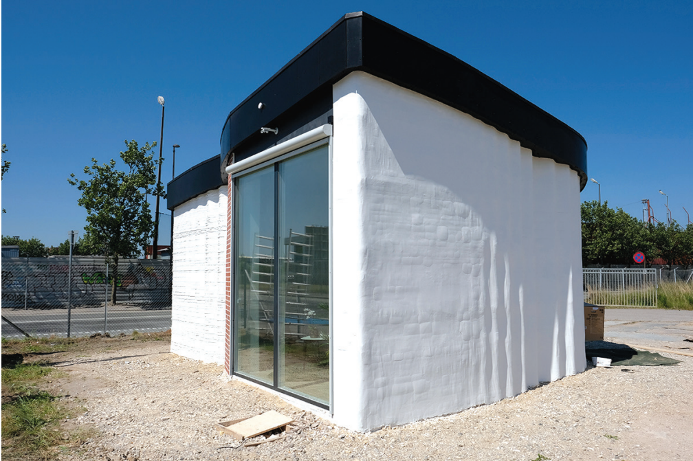
Fig. 4. A printed building completed in 2018 in Denmark by the COBOD company [11]
