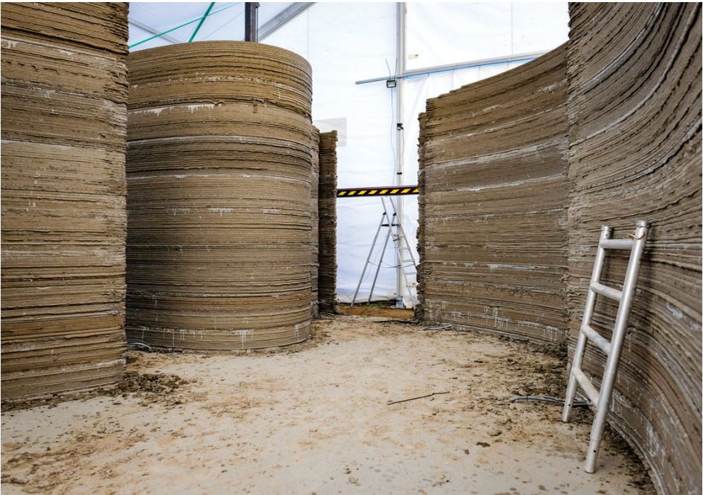
Fig. 5-6. The next phases of building printing – by Cobod [11]
