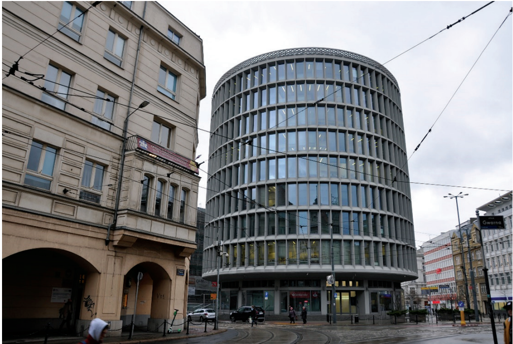
Fig. 3. 'Okraślak' – former department store in Poznań [by author]
