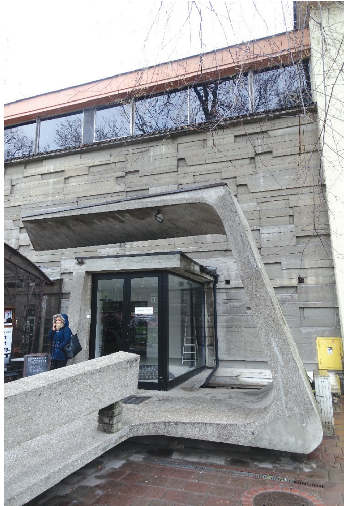
Fig. 4. 'Bunkier Sztuki' Gallery of Modern Art building in Krakow [by author]
