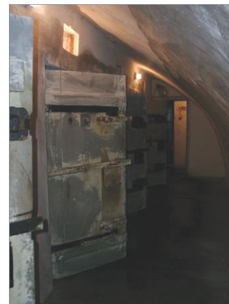
Fig. 6. Former prison in Kielce, interior [27]
