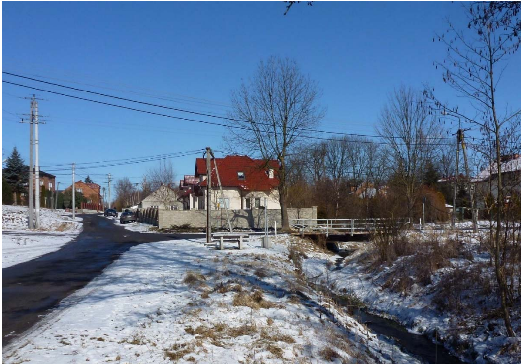
Figure 5. Green corridor in the reality – in the background a bridge over the Bibiczanka river; along the waterway to the left - a narrow carriageway with no space for pedestrians; new residential architecture (in the centre, behind the bridge) with fences close to the bank of the river. Photo: the Author, Bibice, Zielonki commune, 2018.
