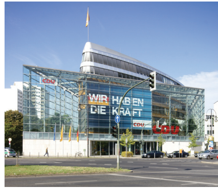
Fig. 2. CDU headquarters in Berlin (arch. Petzinka and Partners, 2001)
