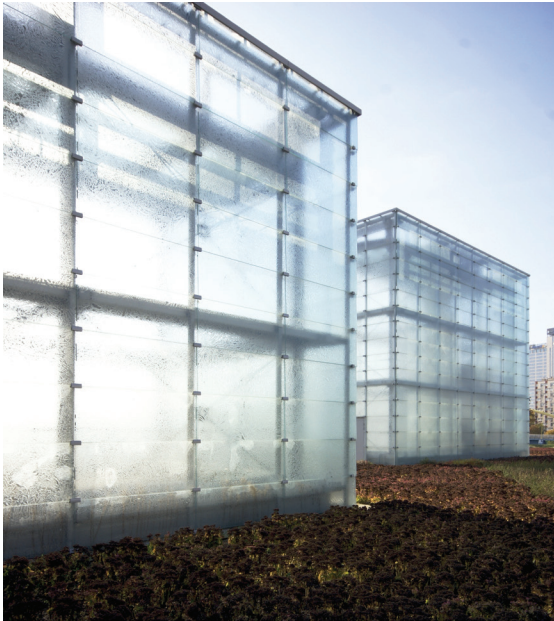
Fig. 6. Silesian Museum in Katowice (arch. Pysal Ruge Architekten, 2013)
