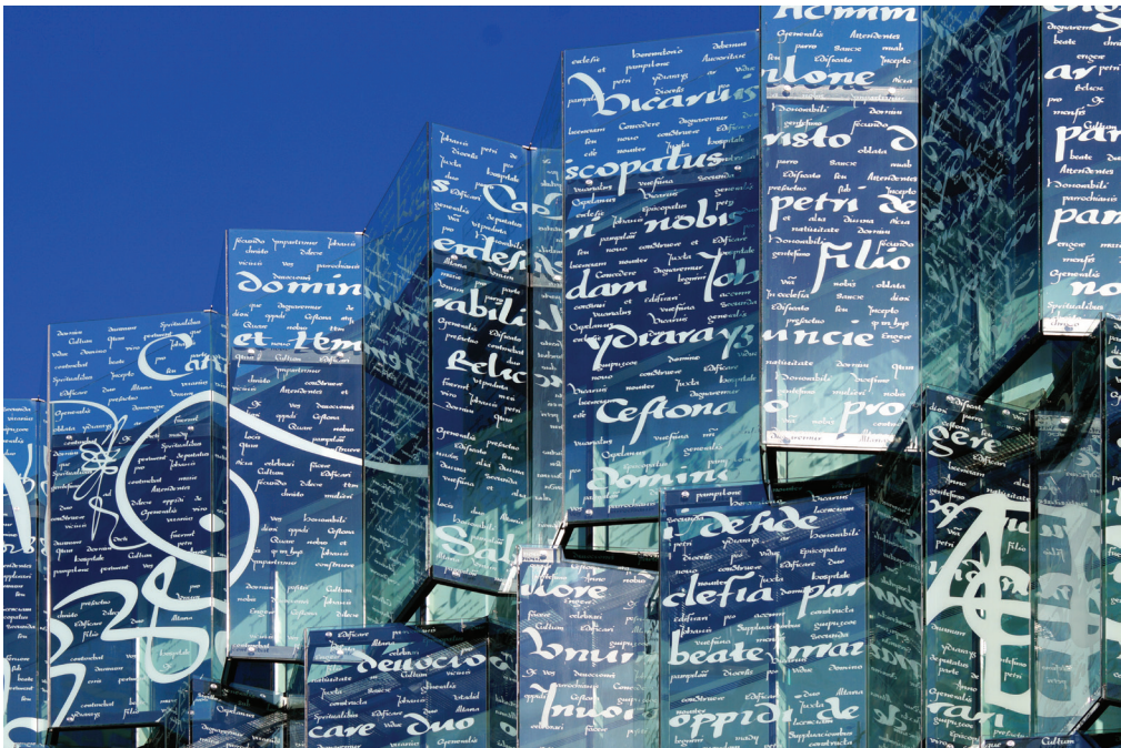
Fig. 27. The example of the façade falling into multiplied types and sub-trends: irregularly serrated and obstructed transparency – Historical Archive of the Basque Country (arch. ACXT, 2013)
