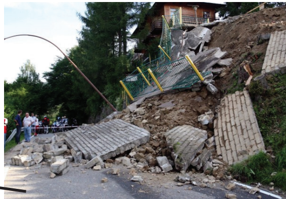
Fig. 2. Landslide on national road No. 87, 28 June 2009 [26]
