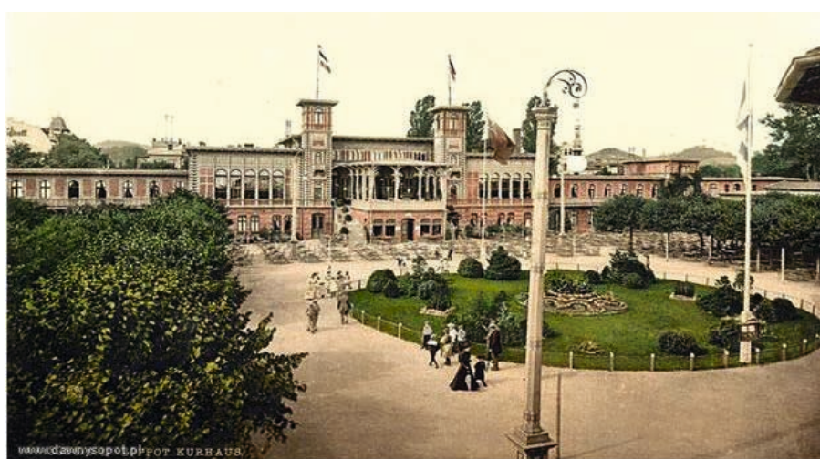
Fig. 3. The Second Spa House, a photograph from ca. 1890 (source: www.dawnysopot.pl )
