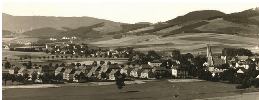
Fig. 22. View of cooperative buildings in the western part of Ludowa Street in Biały Kamień; Weißstein – one of the municipal housing estates erected in cooperation with the „Schlesische Heimstätte”. MWH 2881 (photo, 1930s)
