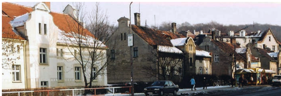
Fig. 1. „Settlement of Four Houses”; Vierhäuser in Wałbrzych; Waldenburg (photo by author)
