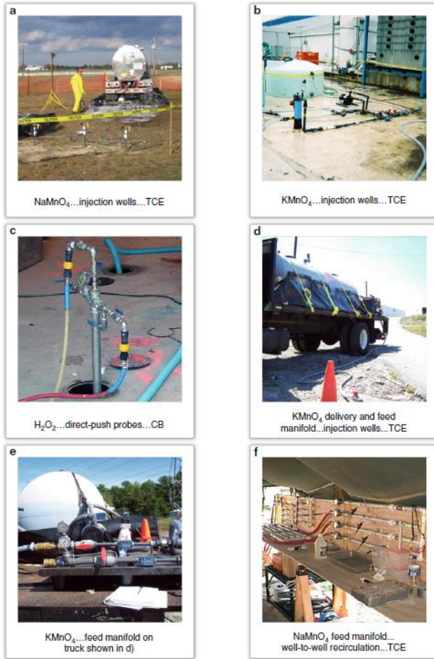
Figure 1.11. Photographs illustrating some of the conditions and infrastructure at sites where ISCO has been deployed for groundwater remediation. Image captions give oxidant used, delivery method, and target contaminants. Note: CB - chlorobenzene, MGP - manufactured gas plant.
