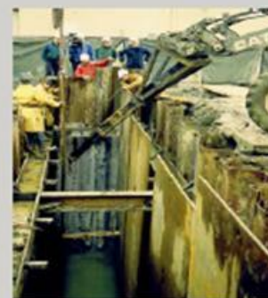
Cofferdam (30 ft, 9 m)
