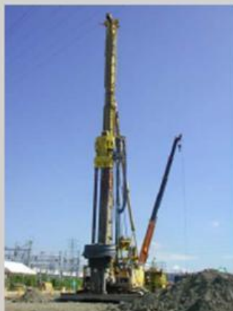
Soil mixing (40 ft, 12 m)
