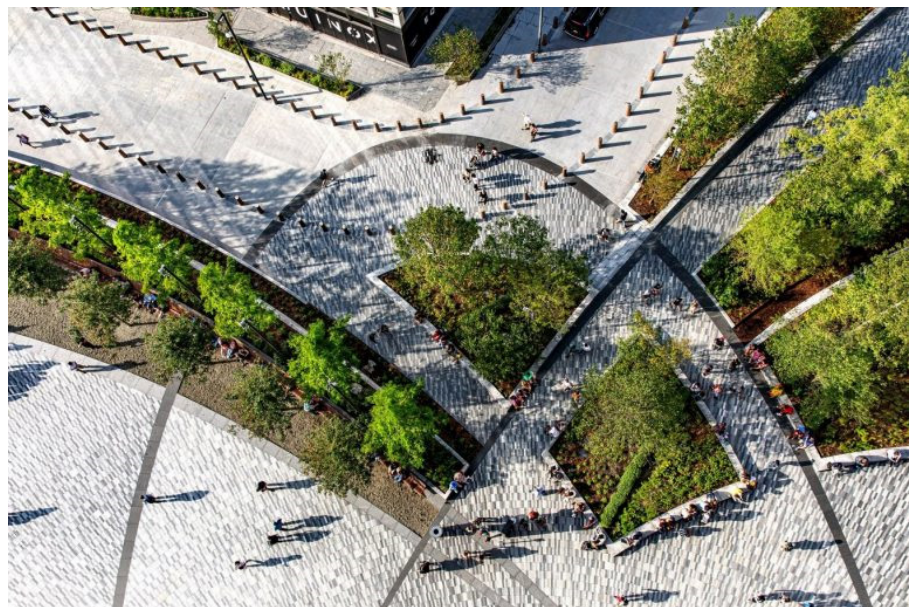
Fig. 45. Detail of the ellipse in the floor plane (source: https://www.nbwla.com/projects/park/public-square-and-gardens-hudson-yards , date of access: 2021/03/01)
