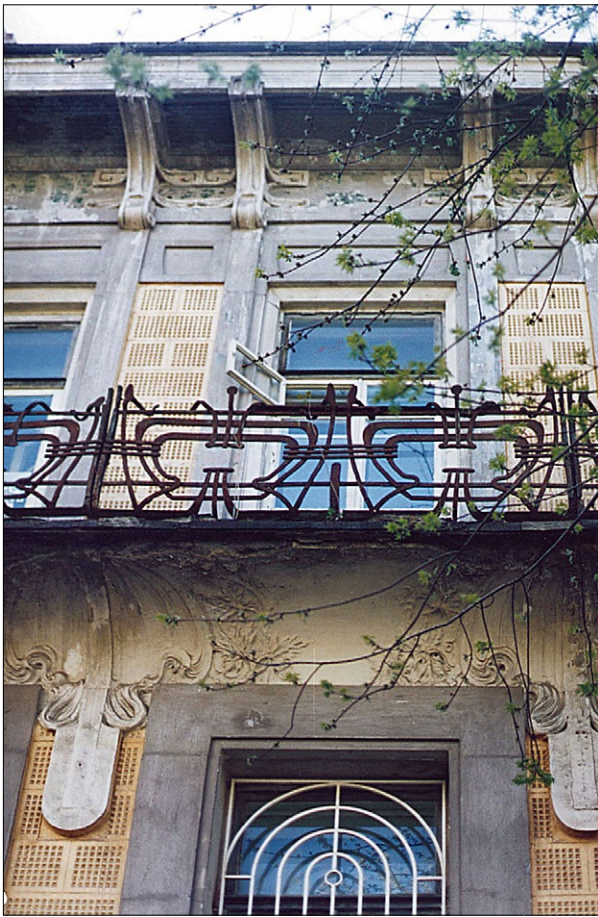
Fig. 6. The Secession style balcony balustrade in the former Kachkovskiy Clinic at 33 Honchara Street in Kyiv, as seen before the restoration; photo by Yu. Ivashko 1999.
