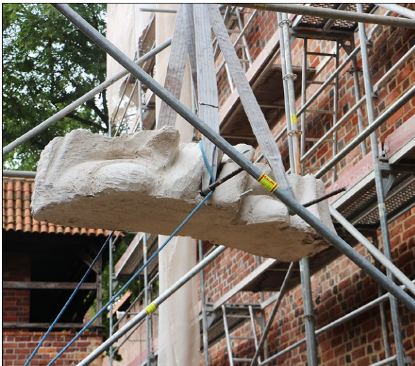
Fig. 9. Transport of the finished segments of the Madonna statue to its place in the outer niche of the presbytery, 2015; photo by L. Okoński.
