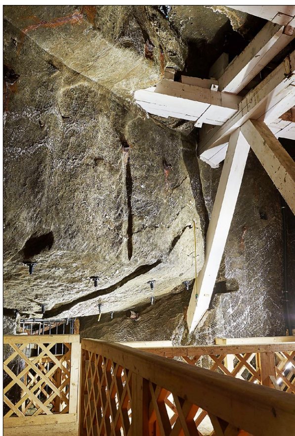
Fig. 3. Wieliczka Salt Mine—reconstruction of truss support in the “Gołuchowski” cavern, using modern anchoring support; photo by AMC.
