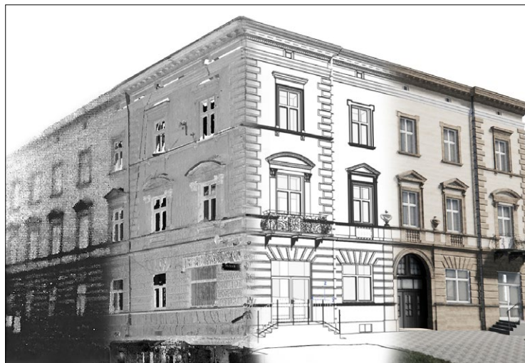
Fig. 1. Comparison of archive photo with the scanning data and HBIM model, from left to right: archival photo, laser scan, linear model view, visualization, photo source: Registration card of architectural and construction monuments no. A-850; by the authors.
