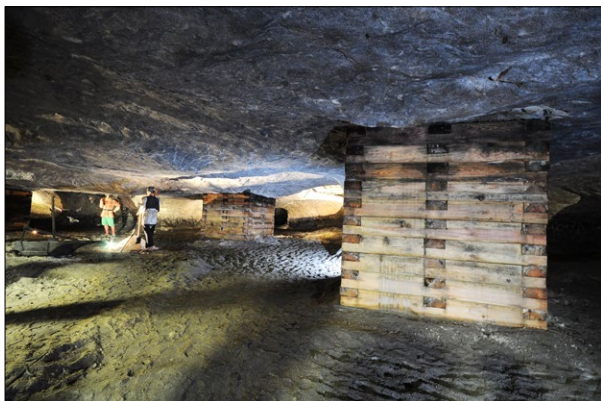
Fig. 1. Sandstone mine in Nagórzycze (Nagórzyckie Grottos)—an example of a modern support structure based on traditional props with cross binding; photo by T. Wieja.
