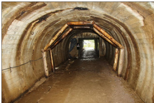
Fig. 2. Podgórze uranium mine in Kowary—conservation works inside the shaft through implementation of polygonal wooden support to the space reinforced and secured with a concrete arched support; photo by T. Wieja.
