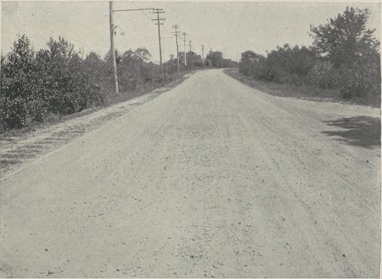
FIG. 71. Effect of Motor-Car Traffic on the Surface of a Broken Stone Road.
