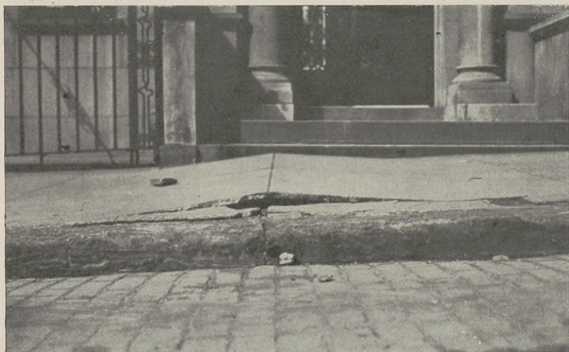
FIG. 177: Bulging of Cement-Concrete Sidewalk, due to Expansion.
