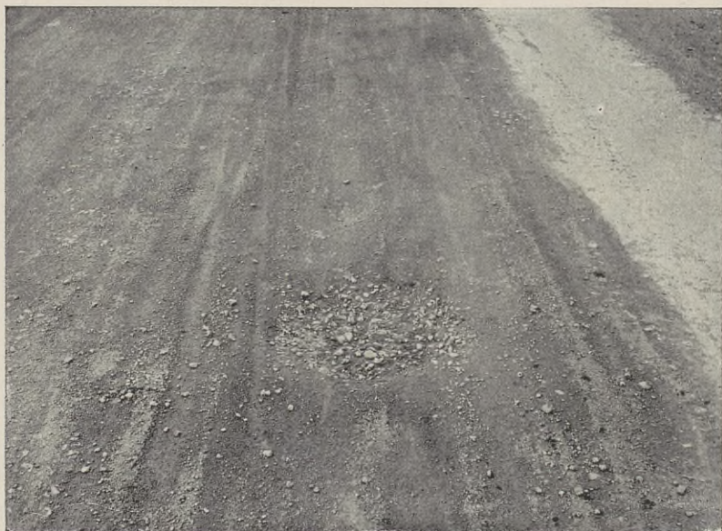
FIG. 73. Pot-hole in the Surface of a Broken Stone Road.
