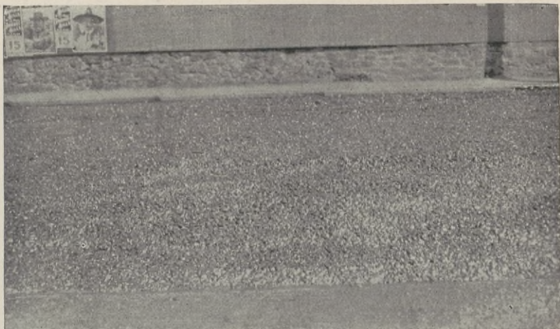
FIG. 102. An Illustration of Uneven Distribution of Bituminous Material.
