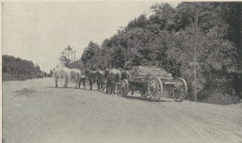
FIG. 7. Heavy Load of Stone on 3-inch Tires.
