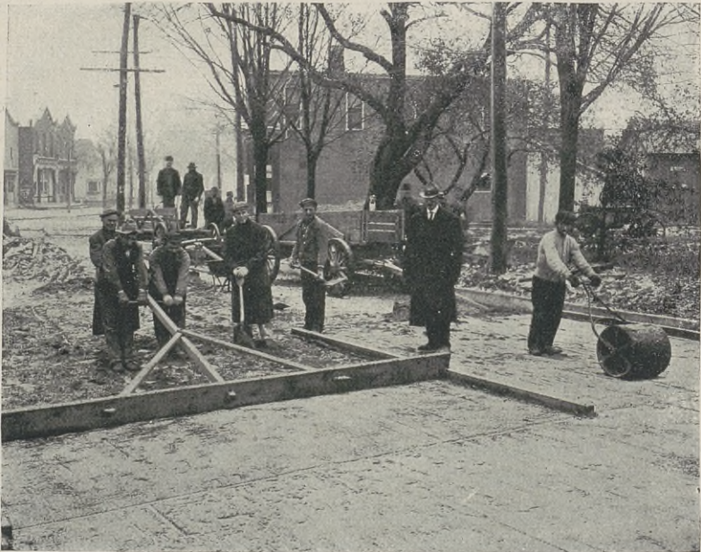
FIG. 146. Smoothing off the Sand Cushion.
