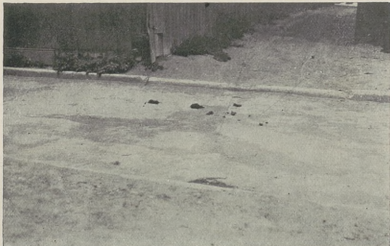
FIG. 138. Uneven Wear of a Cement-Concrete Pavement.
