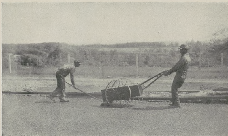
FIG. 111. Application of Seal Coat on Wearing Course of Bituminous Concrete, Class 1. A., with Hand-drawn Distributor and Squeegee.
