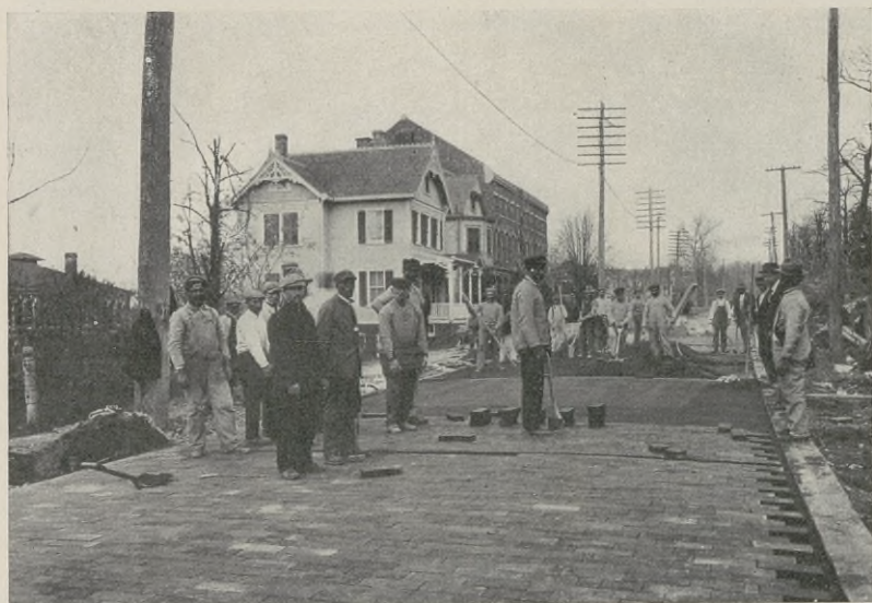
FIG. 117. Construction of Asphalt Block Pavement.
