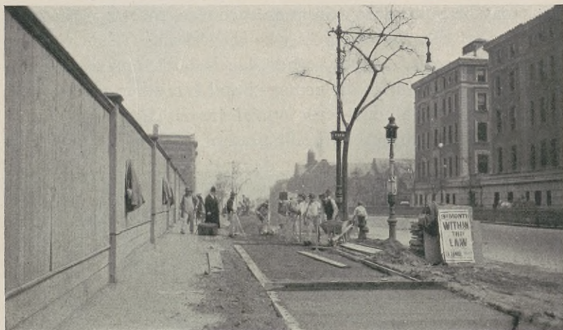
FIG. 175. Straight-Edge Used in Construction of Cement-Concrete Sidewalks.
