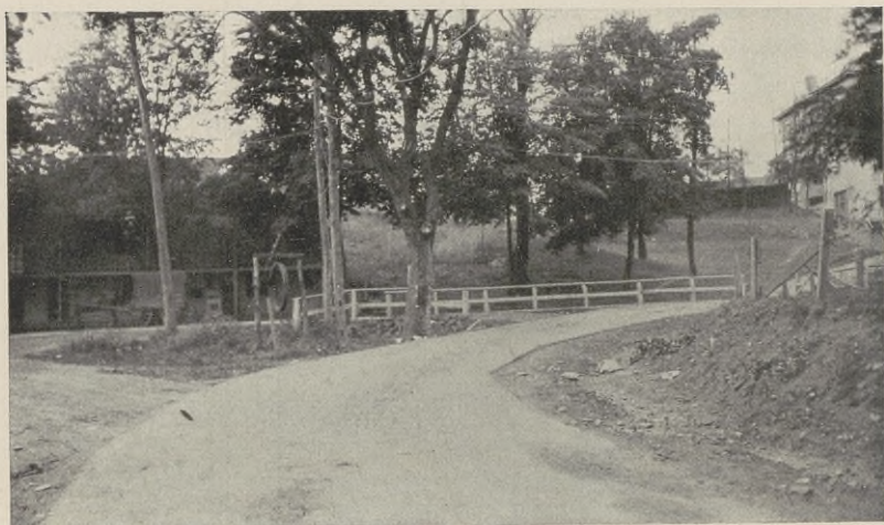
FIG. 27. Example of Poor Curve Design.
