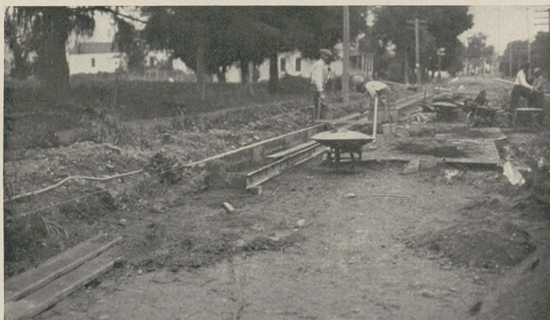
FIG. 181. Metal Form Used in the Construction of a Cement-Concrete Curb and Gutter.
