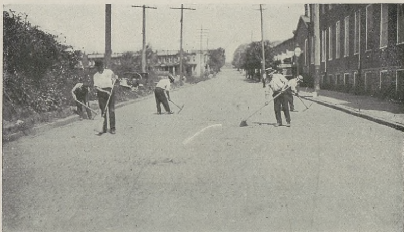
FIG. 154. Cleaning Joints Prior to Application of Bituminous Material.
