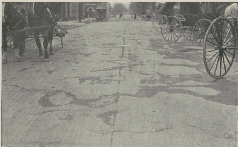
FIG. 137. Failure of a Bituminous Surface on a Cement-Concrete Pavement.
