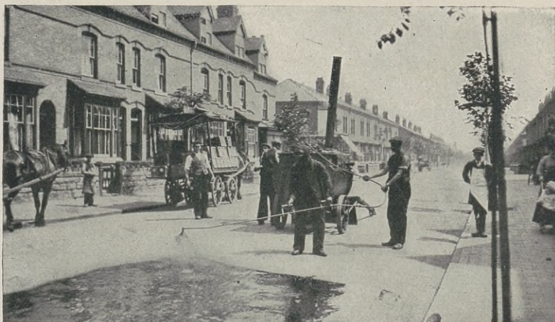
FIG. 87. English Hand-drawn Pressure Distributor.
