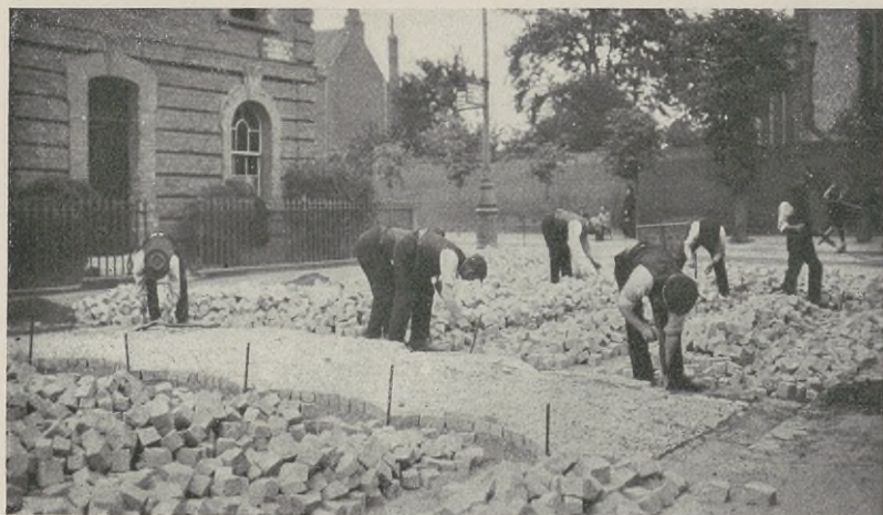
FIG. 159. Construction of a Durax Pavement near London.
