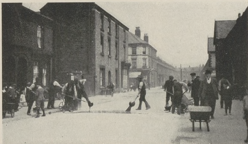
FIG. 98. Construction of "Pitchmac" Pavement in Liverpool.
