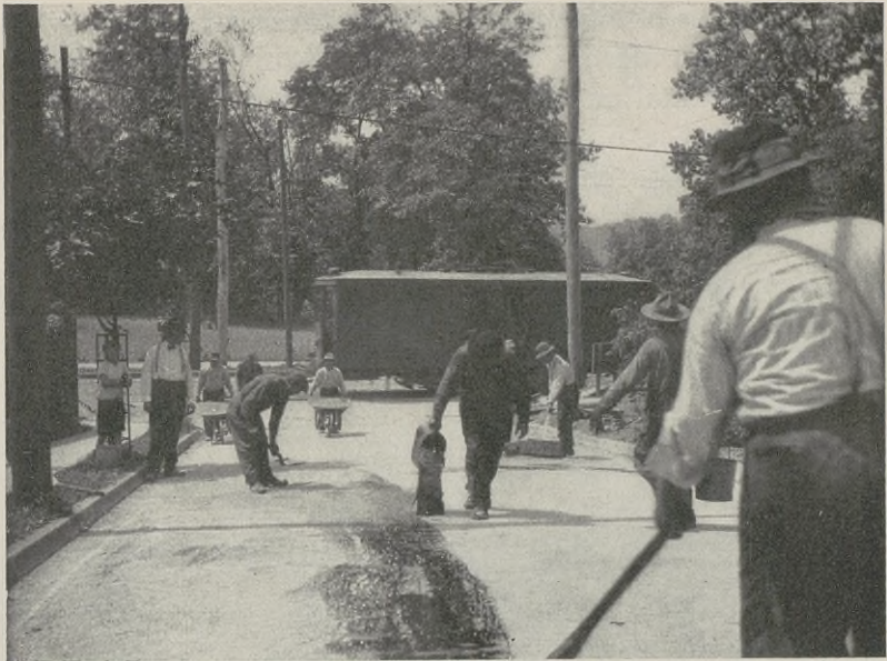
FIG. 110. Application of Seal Coat on Wearing Course of Topeka Bituminous Concrete with Pouring Can and Squeegee.
