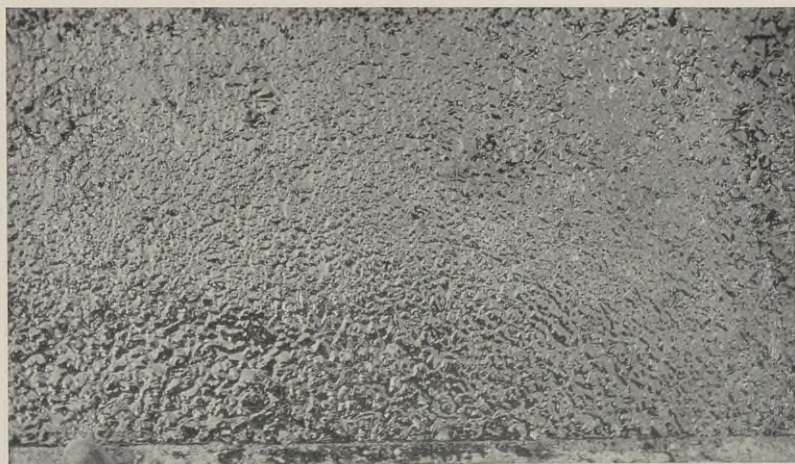
FIG. 112. Surface of Seal Coat on Wearing Course of Bituminous Concrete, Class I. A., Ashokan Highway, Board of Water Supply of the City of New York.
