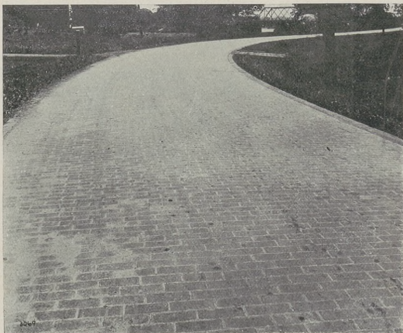
FIG. 151. Cement Grout-filled Wire-Cut-Lug-Brick Pavement on New York State Highway.
