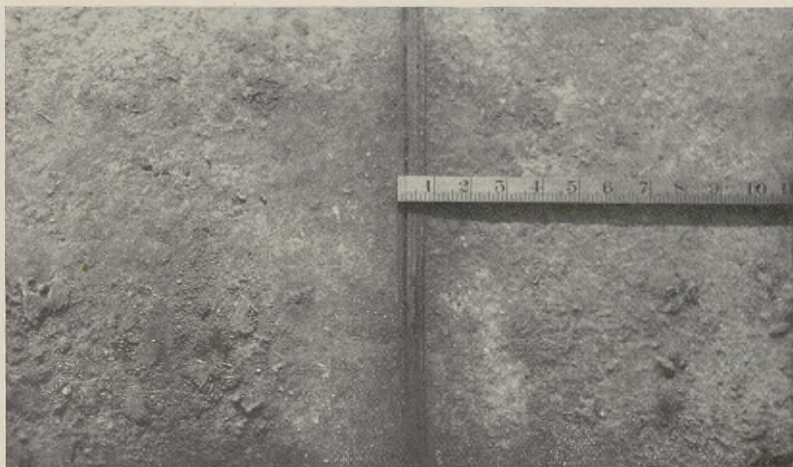
FIG. 133. Expansion-Contraction Joint in Cement-Concrete Pavement.
