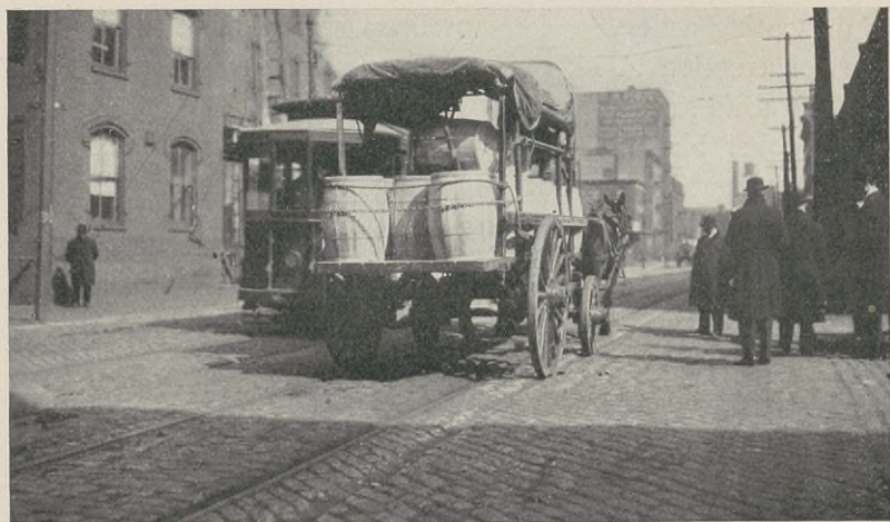
FIG. 9. Wear of Stone Blocks Caused by "Tracking."
