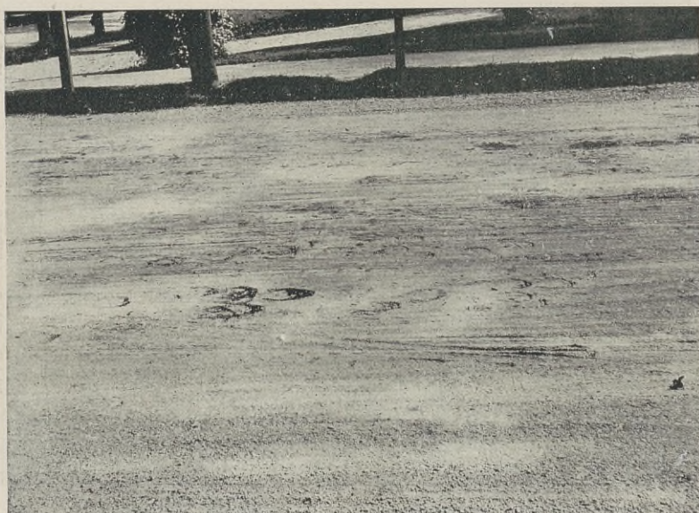
FIG. 93. Failure of Bituminous Surface Due to Using an Excess of Bituminous Material.
