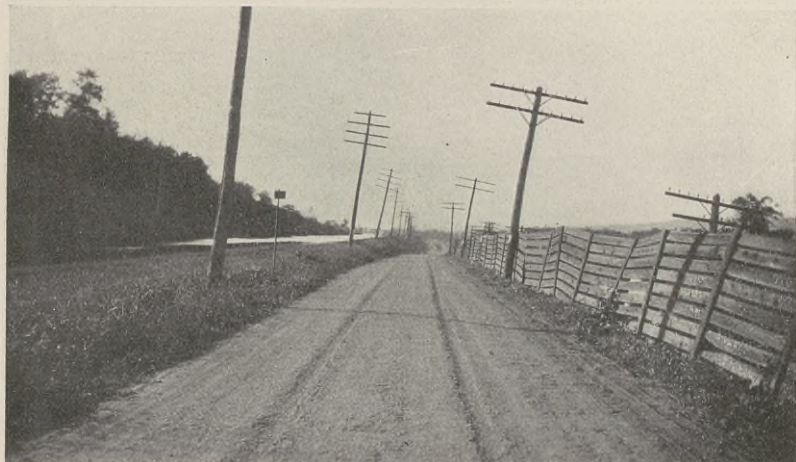
FIG. 8. Ruts Caused by "Tracking."
