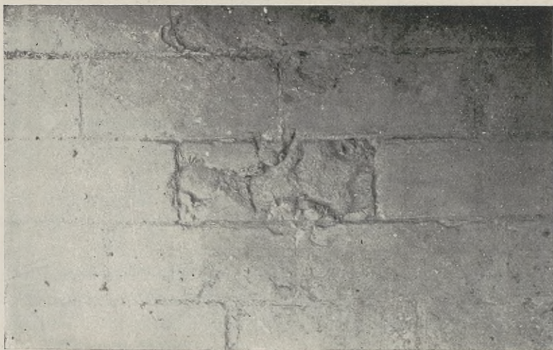
FIG. 148. Poor Brick in a Cement Grout-filled Pavement.
