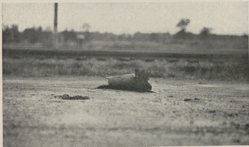
FIG. 92. Failure of Asphaltic Oil Mat Surface Due to Poor Adhesion Caused by Oil Being Applied to Damp Surface.
