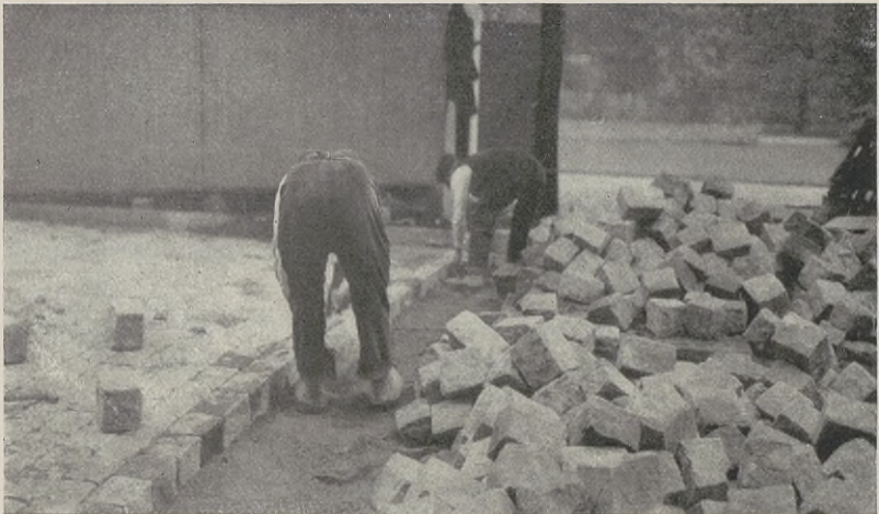
FIG. 157. Construction of Stone Block Pavement in Hamburg, Germany.
