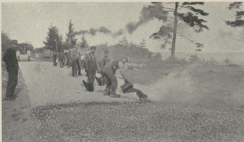
FIG. 101. Example of Uneven Distribution of Bituminous Material.
