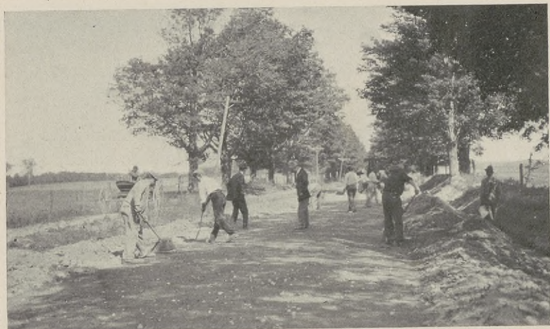
FIG. 97. Voids of Upper Part of Foundation Course Being Filled with Sand.
