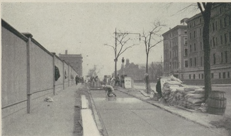
FIG. 176. Use of Float in the Construction of the Surface of Cement-Concrete Sidewalks.
