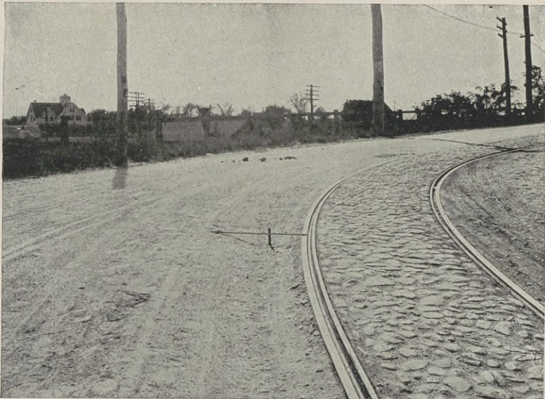
FIG. 72. Wear on the Inside of the Curve Produced by Motor-Car Traffic.
