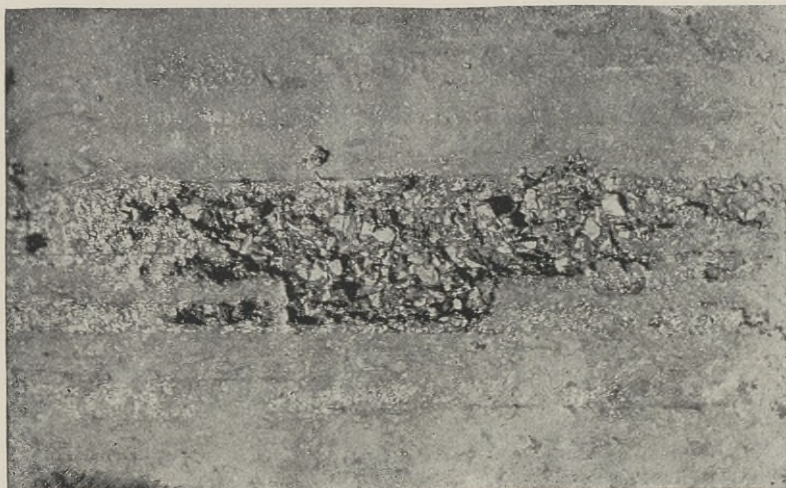
FIG. 125. Soft Seal Coat Torn up Due to Adhesion to Tires.
