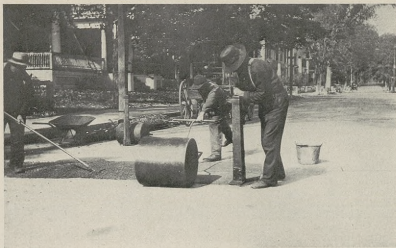
FIG. 123. Repairing a Trench Opening in a Bituminous Concrete Pavement.
