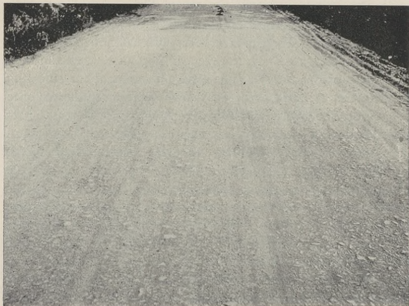
FIG. 70. Mosaic Condition of the Surface of a Broken Stone Road After Binder Has Been Swept Away by Traffic.
