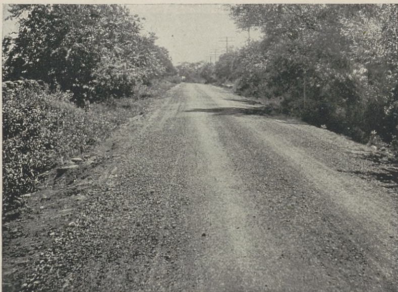
FIG. 124. Result of Using a Poor Grade of Tar.
