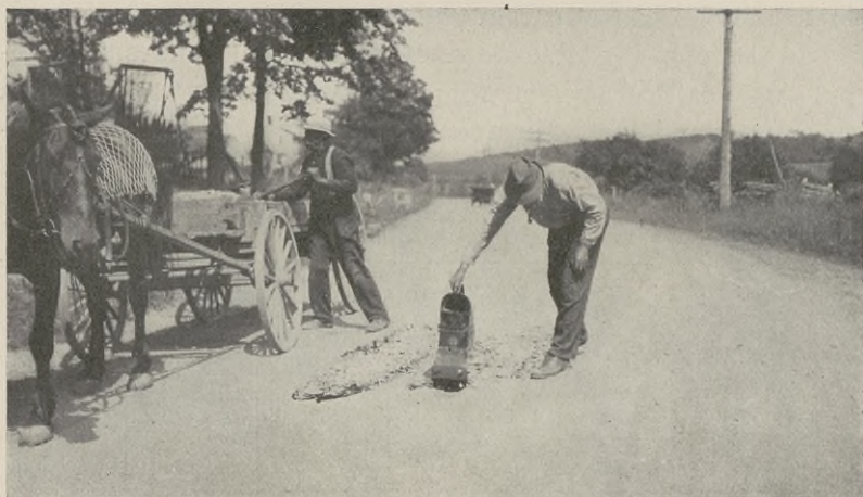
FIG. 99. Improper Method of Repairing Holes. Depressions Filled with Broken Stone and Light Oil.
