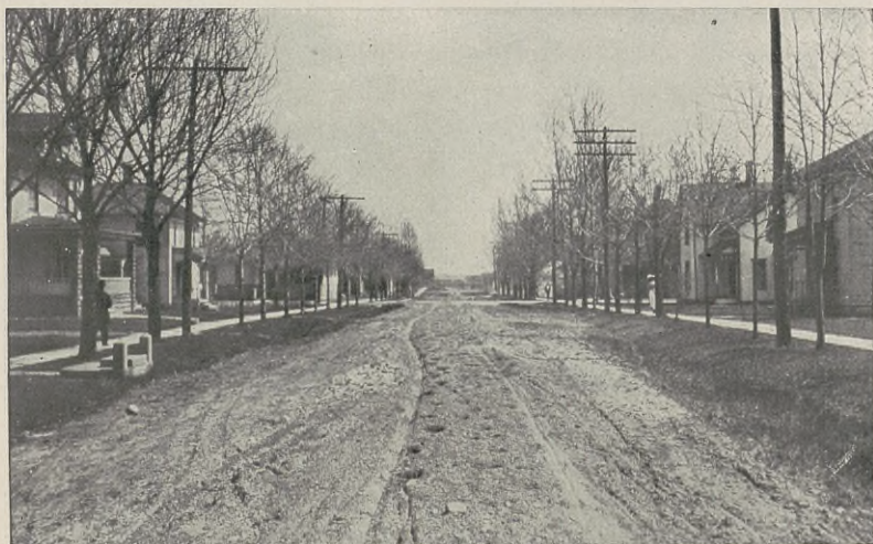
FIG. 55. An Earth Road Under Poor Maintenance.
