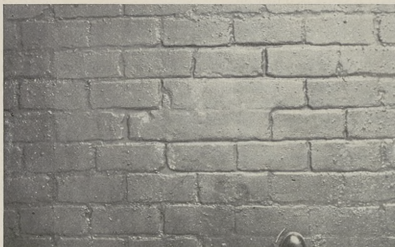
FIG. 149. Chipping Out of Grout Filler in the Joints by Horse-drawn Traffic.
