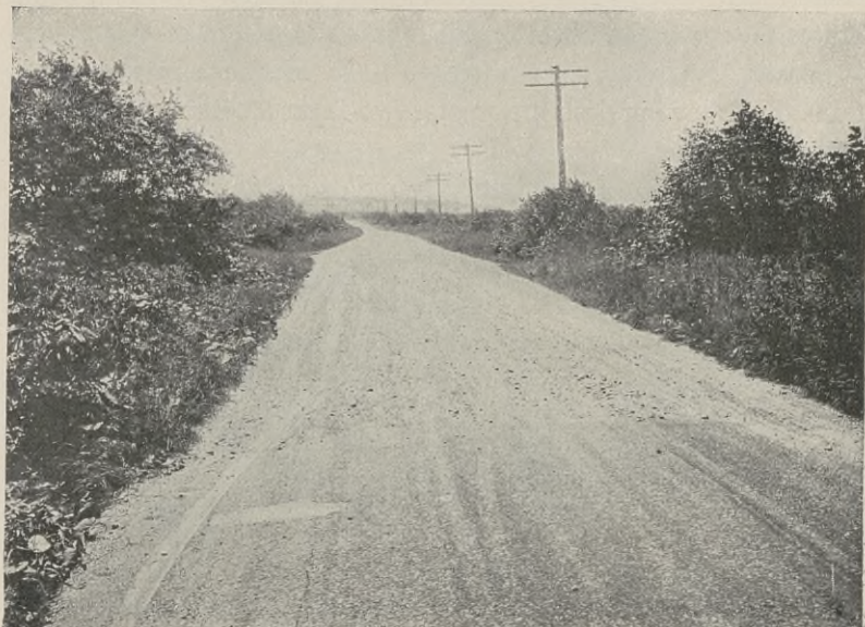
FIG. 107. Upper Part, Water-bound Broken Stone Road. Lower Part, Bituminous Concrete Pavement, Class 1. A., without Seal Coat, Rhode Island State Highway.
