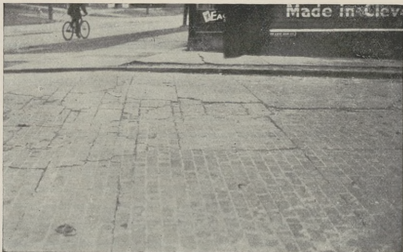
FIG. 144. Result of Constructing a Brick Pavement on a Sand Foundation.
