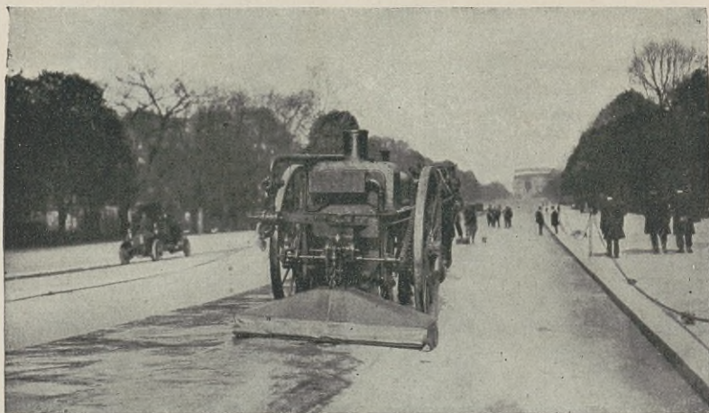
FIG. 90. Hedeline and Voisembert Pressure Distributor. (French Machine.)
