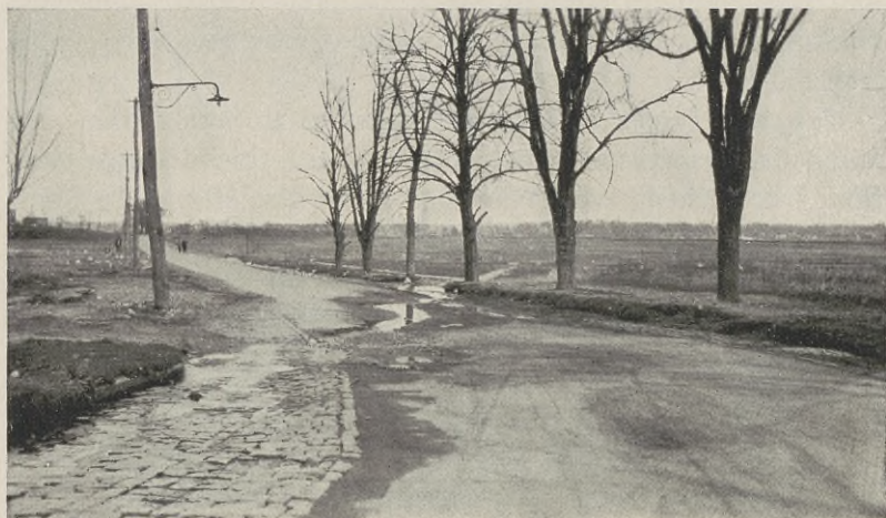
FIG. 185. Location Where Catch-Basin and Culvert Should Have Been Used to Take Storm Water Under the Highway.
