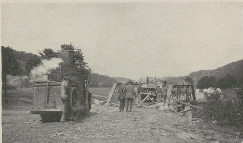
FIG. 135. Rolling Hassam Cement-Concrete Pavement.
