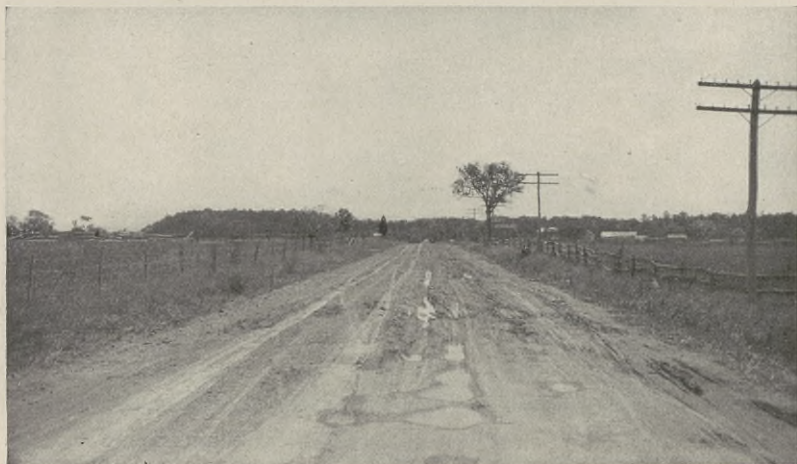
FIG. 104. Result of Using Improper Combination of Bituminous Materials.
