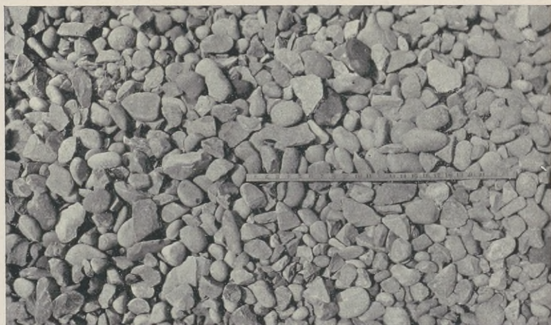
FIG. 57. Lower Course of a Gravel Road Before Being Filled with Fine Material.
