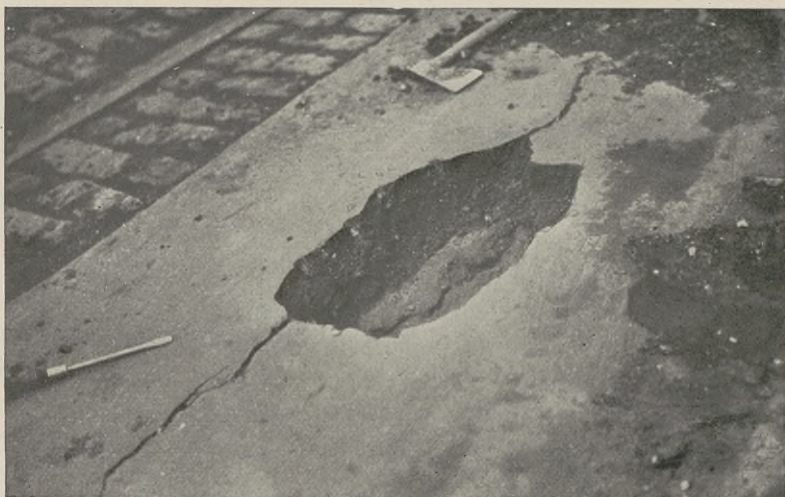
FIG. 128. Crack in Concrete Foundation Due to Poorly Drained Subgrade.
