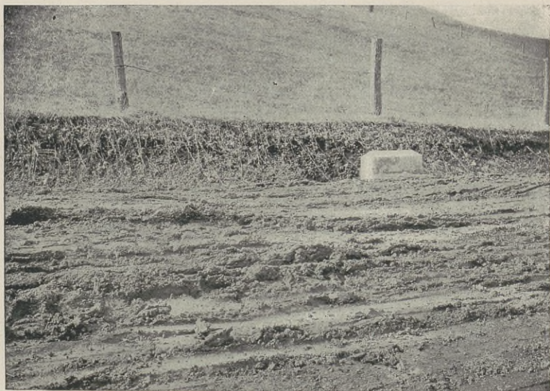
FIG. 103. Surface of Soft Broken Stone and Asphaltic Oil Subjected to Horse-drawn Vehicle Traffic.
