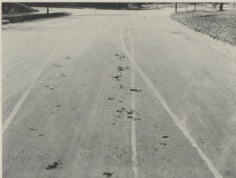
FIG. 94. Calk Holes in a Bituminous Mat Surface.
