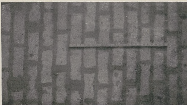
FIG. 155. Surface of Badly Worn Brick Pavement, Showing Condition, After Three Years' Service, of Joints Repaired with Asphalt Filler.
