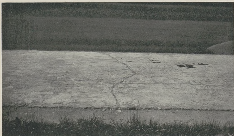
FIG. 132. Crack in Cement-Concrete Pavement Due to Contraction.
