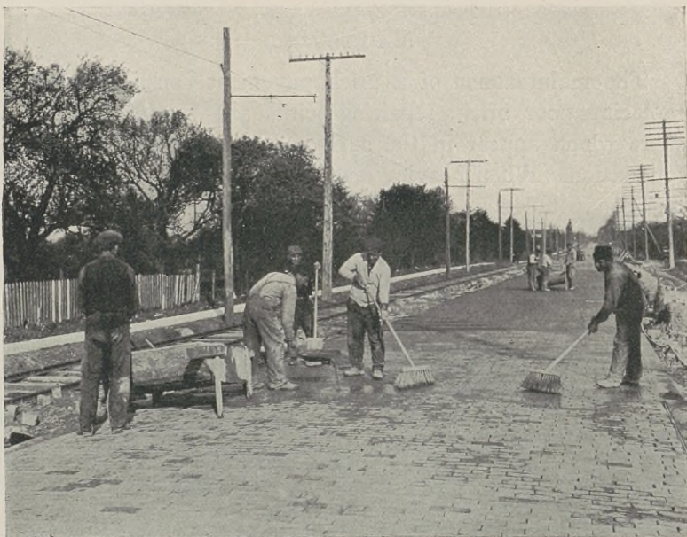
FIG. 152. Application of Cement Grout Filler.
