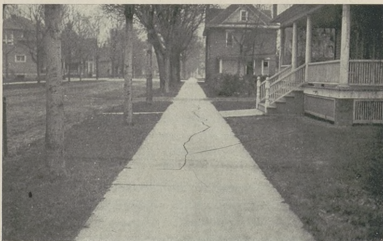
FIG. 178. Longitudinal Crack in Cement-Concrete Sidewalk, due to Frost Action.
