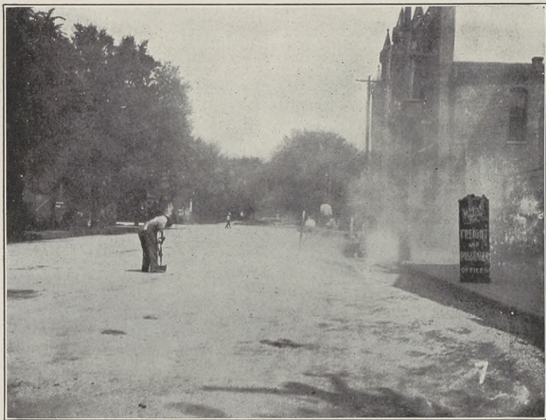
PRELIMINARY SWEEPING IN PREPARATION FOR TARVIA (Jackson, Tenn.).
