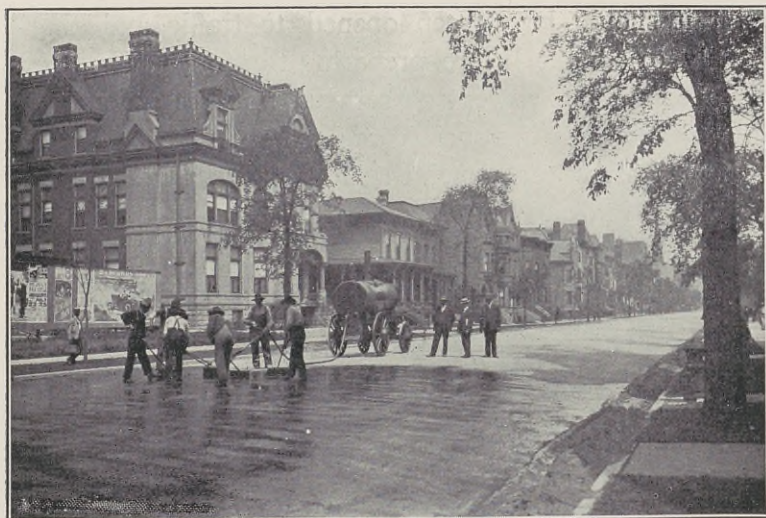
SPREADING BY HOSE FROM TANK. (Michigan Boulevard, Chicago).
