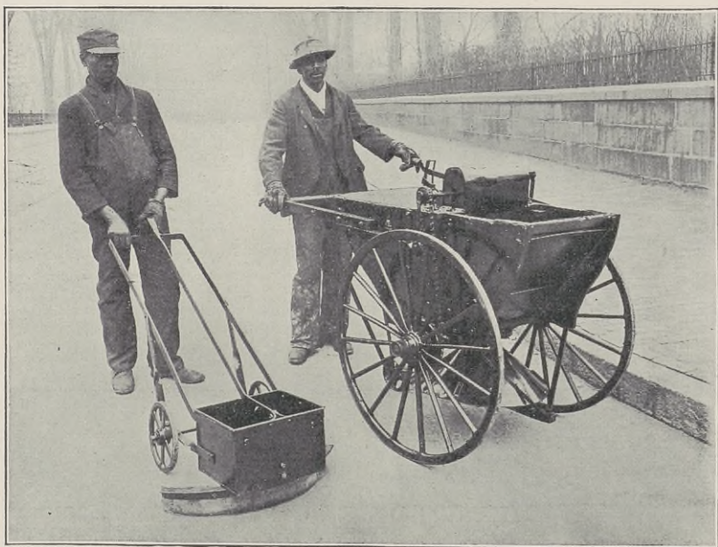
FLUSH COAT SPREADING MACHINE. (Patented.)
