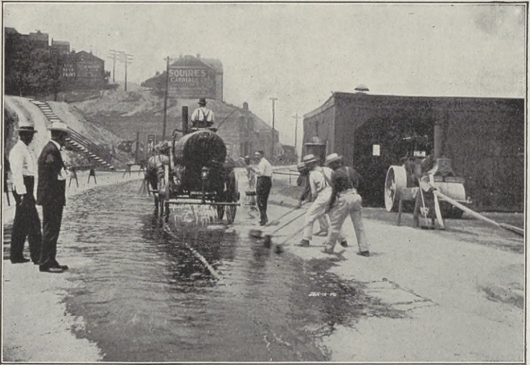
SPREADING TARVIA FROM A SLOTTED SPRINKLER (Pittsburg, Pa.).
