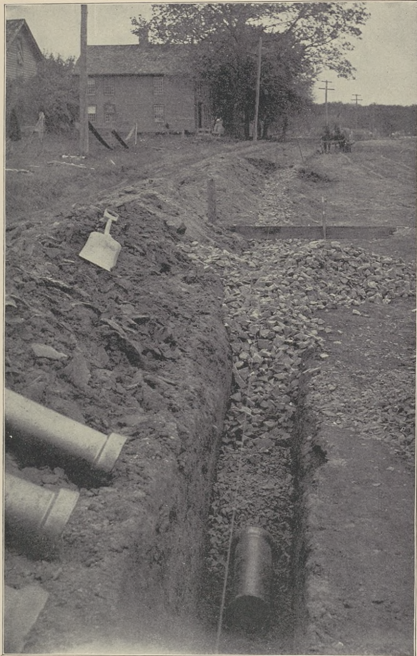
FIG. 18.—Detail of Drain.
