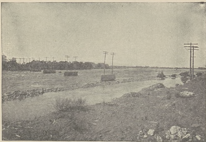
FIG. 86.—Chambly-Montreal Line Crossing the Richelieu River.
