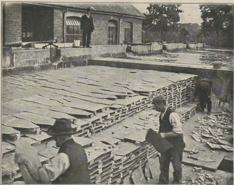
Fig. 30.—Slate Beds at Devizes, Showing Method of Placing Slates in Position.
