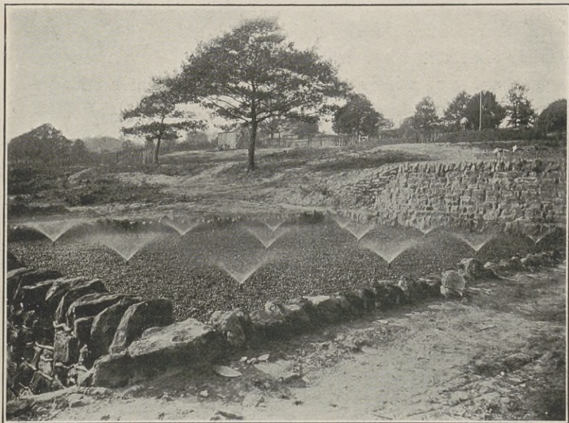
Fig. 49.—Fixed Sprinklers in Operation at Tunbridge Wells.
