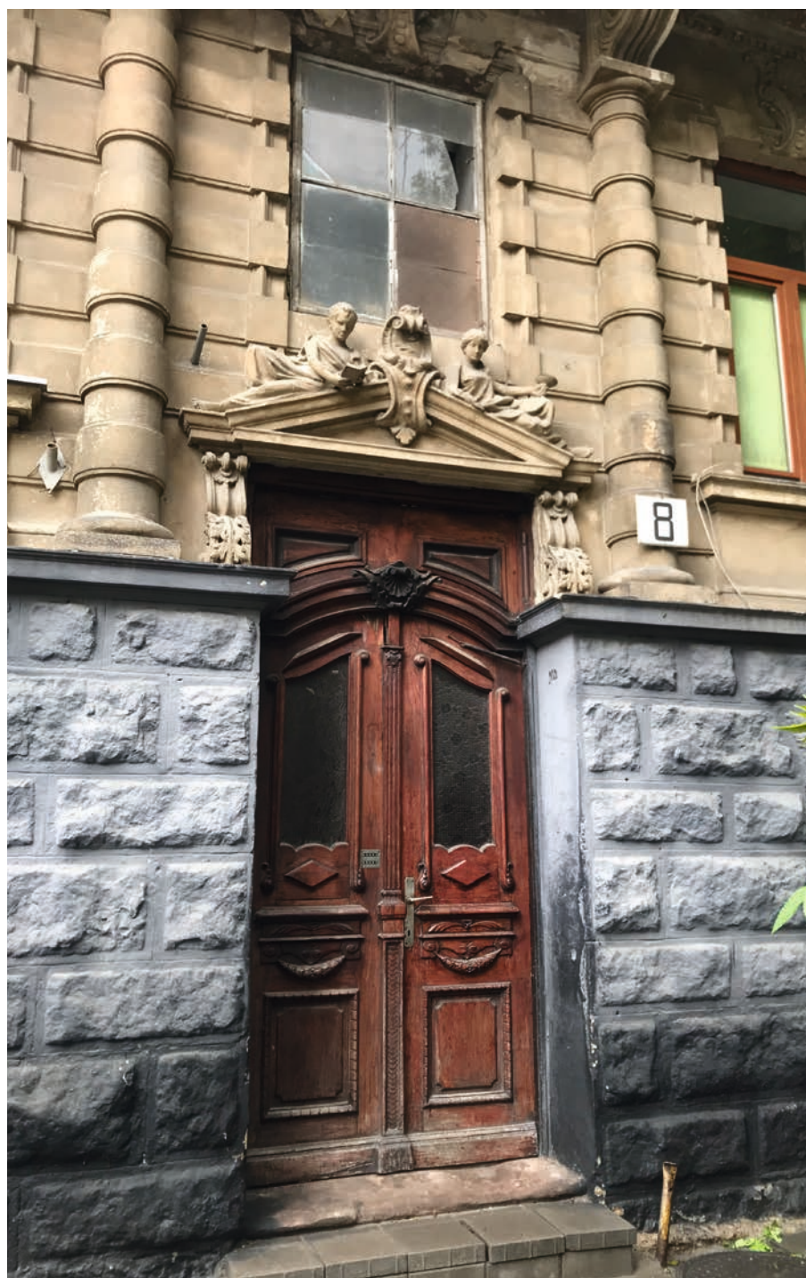
Fig. 4. Decorative solution of the entry door at 8 G. Smolskyi St. in Lviv (photo by author)
