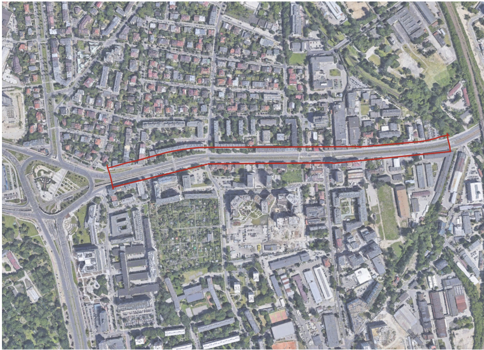
Fig. 7. Mogilska Avenue has four lanes and a tram in the middle. The redevelopment was a chance to reduce car lanes in favour of pedestrian and cyclist comfort (Google Earth, n.d.)
