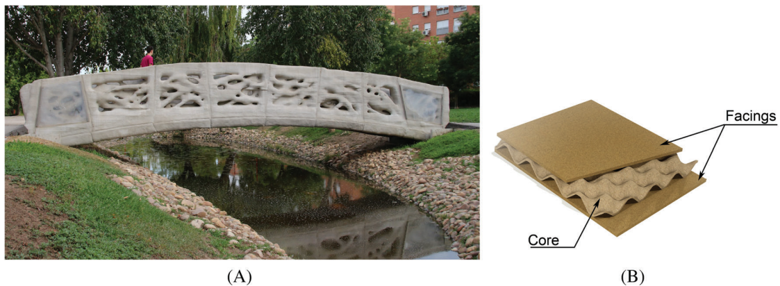
FIGURE 1 Examples of sophisticated microstructures: The first in the world 3D printed concrete bridge in Madrid, Spain (A) and a light layer sandwich panel with a dual corrugated high-density fiberboard core (B)
