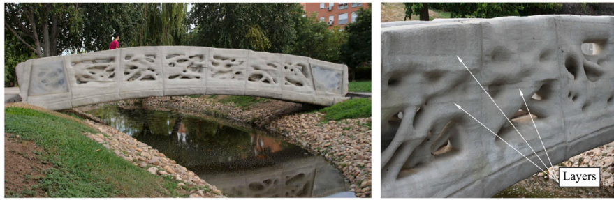
Fig. 1. Example of sophisticated mesostructure achieved through additive manufacturing: a concrete 3D printed bridge in Madrid, Spain.
