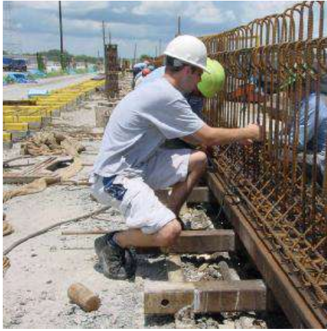
Fig. 2.5: Reinforcement installation [Choi, 2006]
