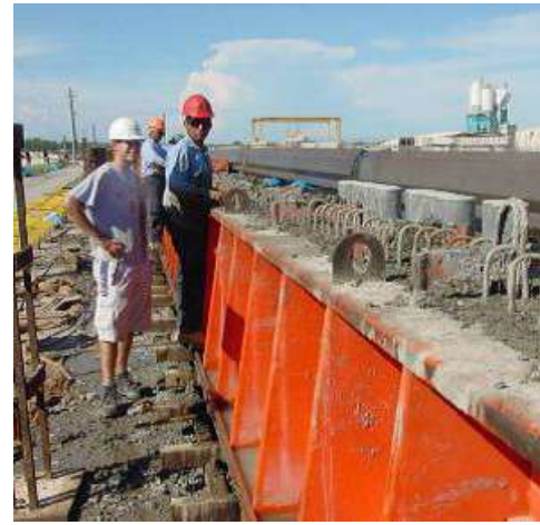
Fig. 2.6: Casting of concrete [Choi, 2006]
