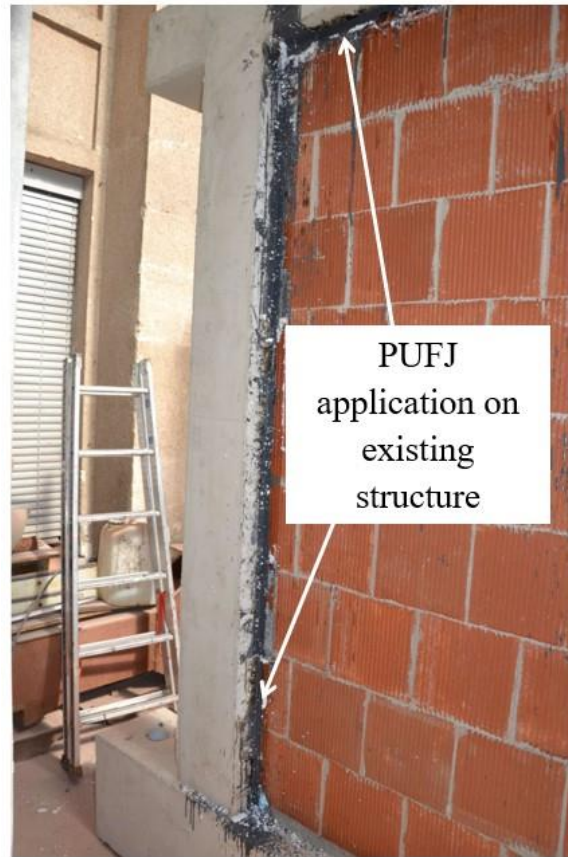
Figure 4.17. PUFJ application on the Frame B.
