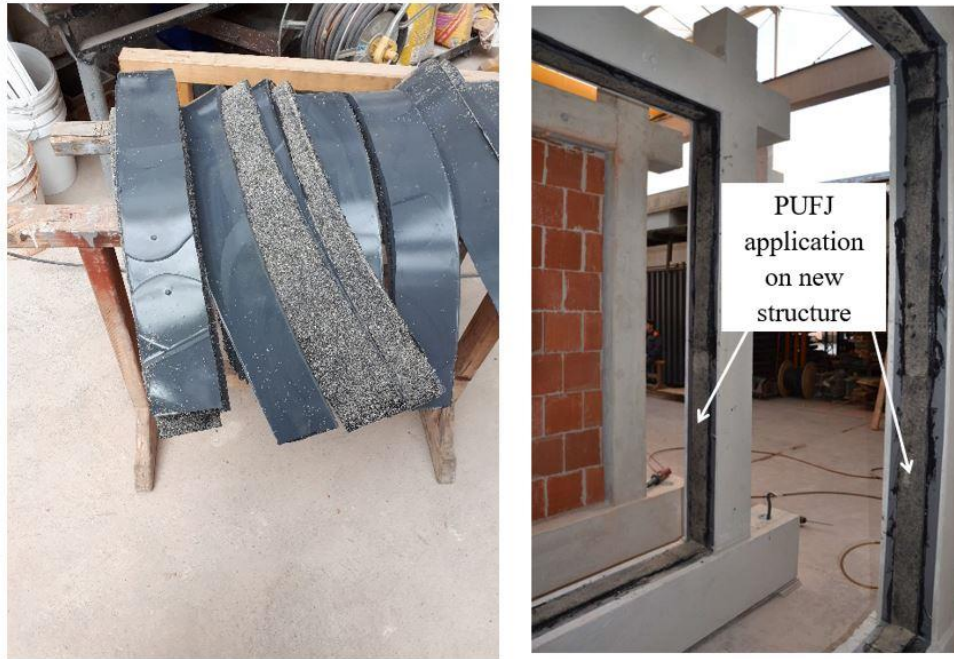
Figure 4.18. Prefabricated PUFJ laminates (left) and application on the Frame C (right).
