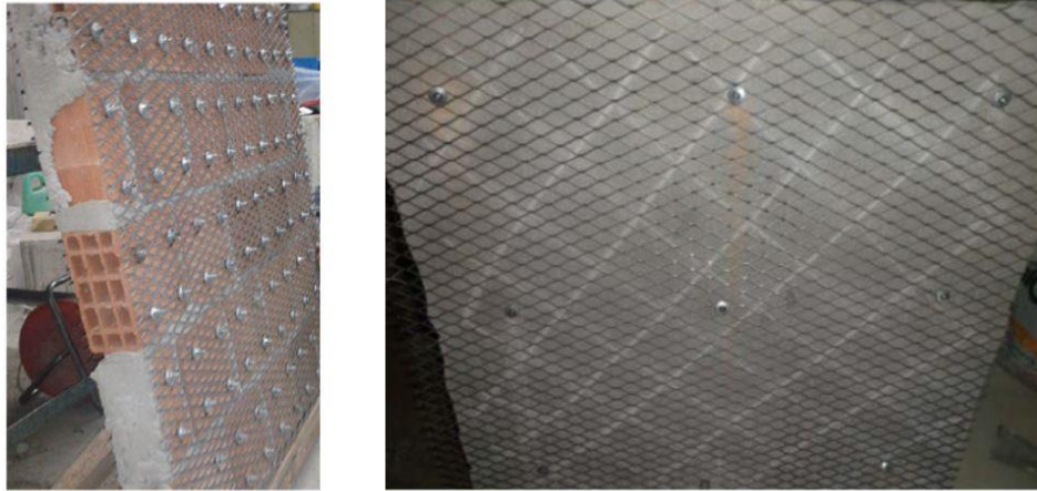
Figure 3.41. Steel mesh installation (left) [adapted from Cumhur et al. (2016)] and ferrocement panel (right) [adapted from Leeanansaksiri et al. (2018)].
