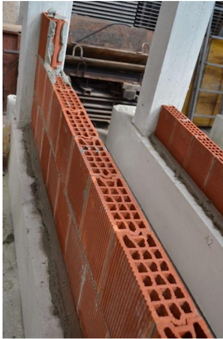
Figure 4.14. Brick blocks arrangement in the frame.
