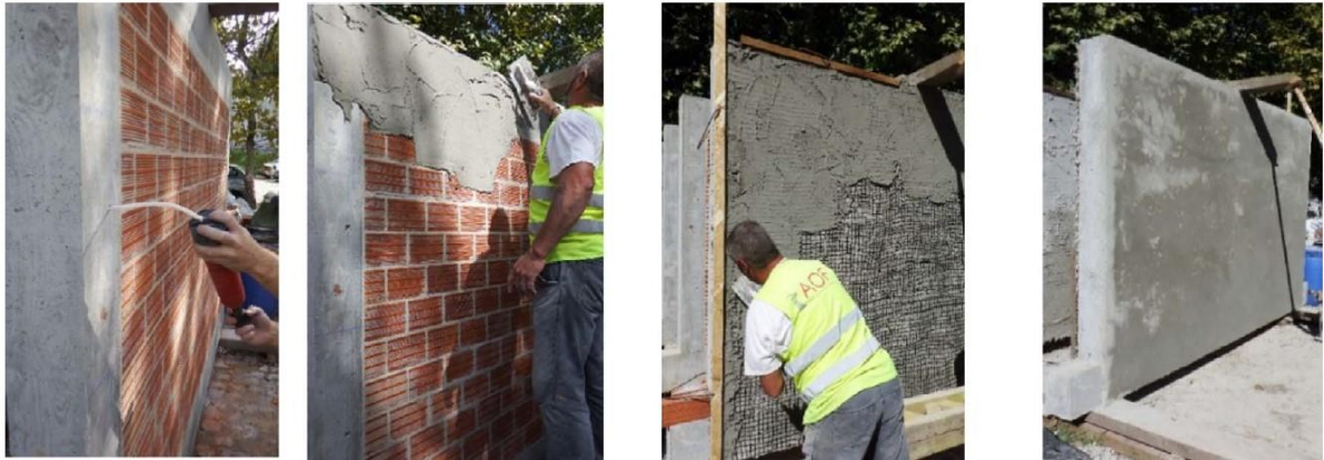
Figure 3.42. Step by step TRM application on the wall [adapted from Akhoundi et al. (2018)].
