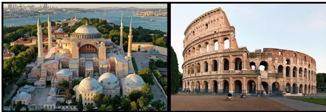
Figure 1.1. Ancient great masonry buildings; Hagia Sophia (left) [Anadolu Agency] and Colosseum (right) [Wikipedia].
