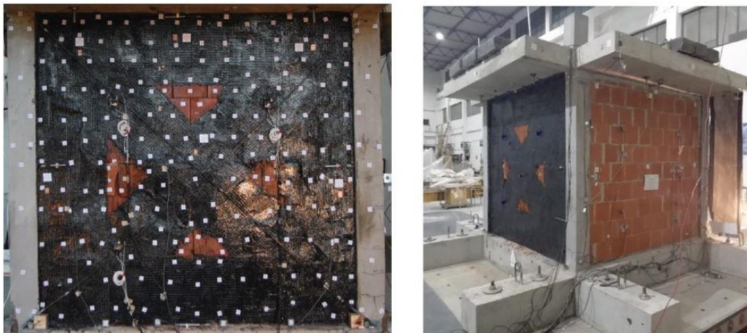
Figure 4.50. FRPU intervention on Type B infills; front (left) and perspective (right) views.
