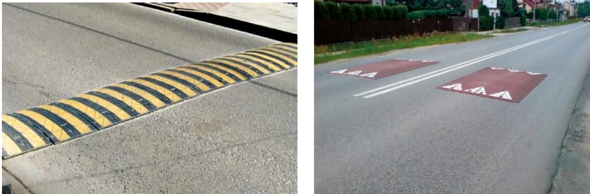
Figure 22: Examples of the vertical deflections: speed hump (left) and speed cushion (right), source: [157]
