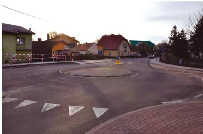
Figure 23: Example of the intersection related measure: mini roundabout. Source: [157]
