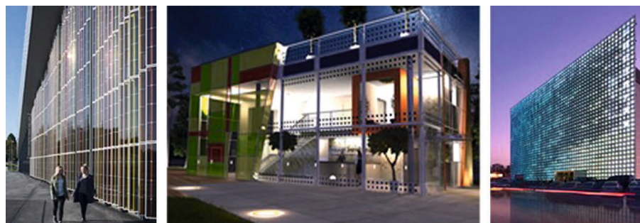
Fig. 5. Artistic effect potential created by BIPV: left – coloured PV façades made of 3rd generation PV cells-Swiss Tech Convention Centre (photo by Swiss Tech Convention Centre); middle – semitransparent a-Si modules in Copper solar house (author's collection); right – interactive PV-LED façade of the Xicui Entertainment Hall (photo by Simone Giostra©)
