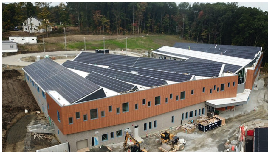
Fig. 9. Shaping of the building's form with the use of roof PV shades in Annie E. Fales Primary School building (photo HMFH Architects©)
