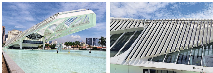
Fig. 6. BIPV in the Museum of Tomorrow as a "supplementary" element of aesthetic function (photo from author's collection)
