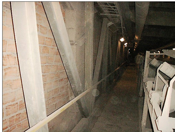
Fig. 4. Interior reinforced concrete flyover, 2008; photo by D. Bajno
