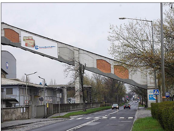
Fig. 3. View of the reinforced concrete flyover, 2022; photo by Ł. Bednarz
