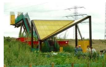
Il. 1.6. Between the Waters: The Emscher Community Garden. Autonomous water treatment system. Instalacja artystyczna na Emscherkunst.2010 i Emscherkunst.2013, autor: Marjetica Potrč and OOZE: Eva Pfannes, Sylvain Hartenberg (fot. Shilesh Harihara, 2010)
