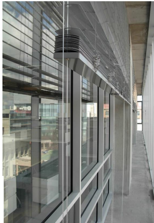
Figure 22. Double wall and controlled blinds. Source: W.Kujawski
