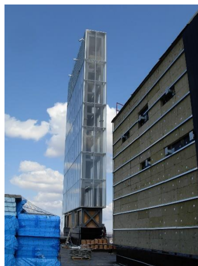
Figure 21. Solar chimney on the roof. Source: W. Kujawski
