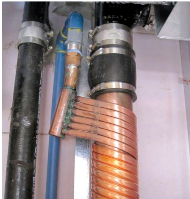
Figure 10. Drainwater heat recovery Source: l'OEUF
