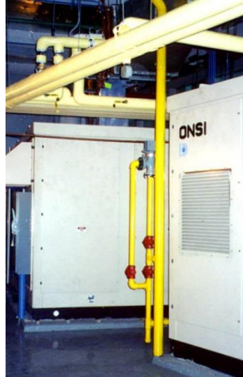
Figure 28. Fuel Cells. Source: W.Kujawski
