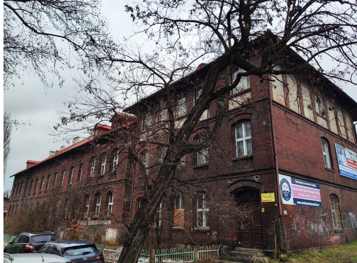
Ill. 1. The building at 2 Londzina Street, October 2021. Photo J. Świerzawski
