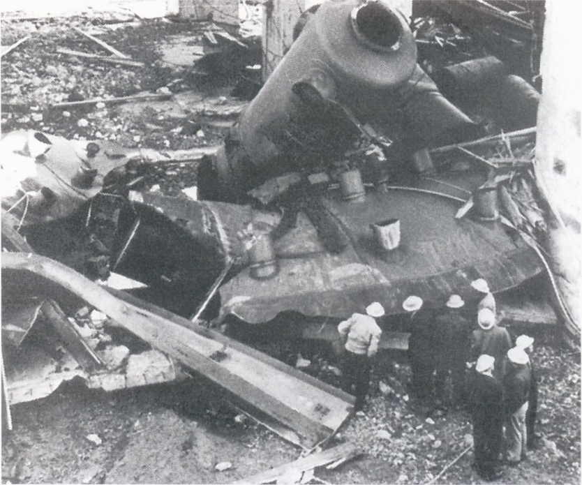
Fig. 5. Some fragments of the failed torispherical head
