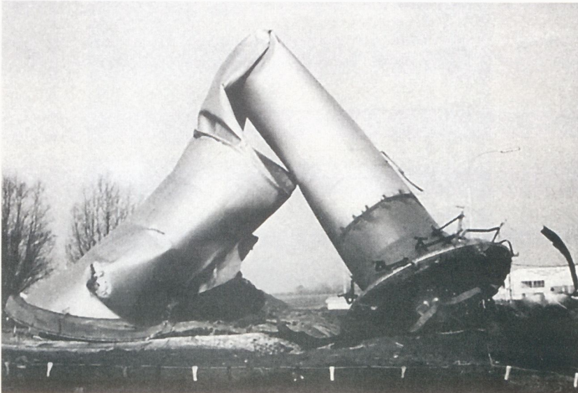
Fig. 8. The failed water tower (which collapsed after being filled with water for the first time)
