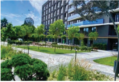
III. 7. Tiffany housing development, 80a Pasichna Street (Lviv), completed in 2022 Photograph by: B. Cherkes
