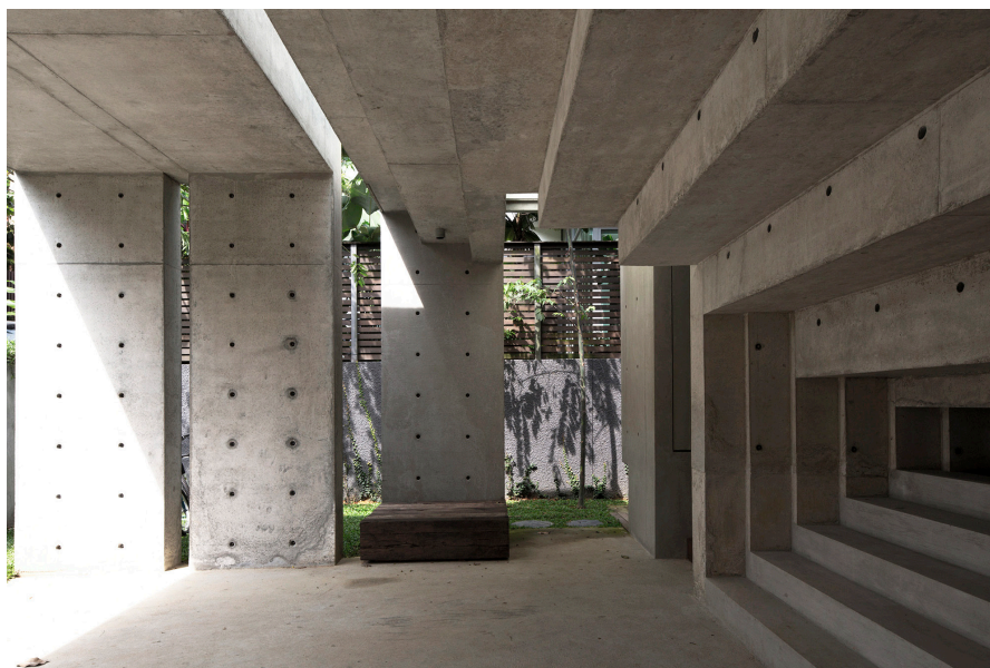
II. 4.51. Channg Architects, Namly House .
