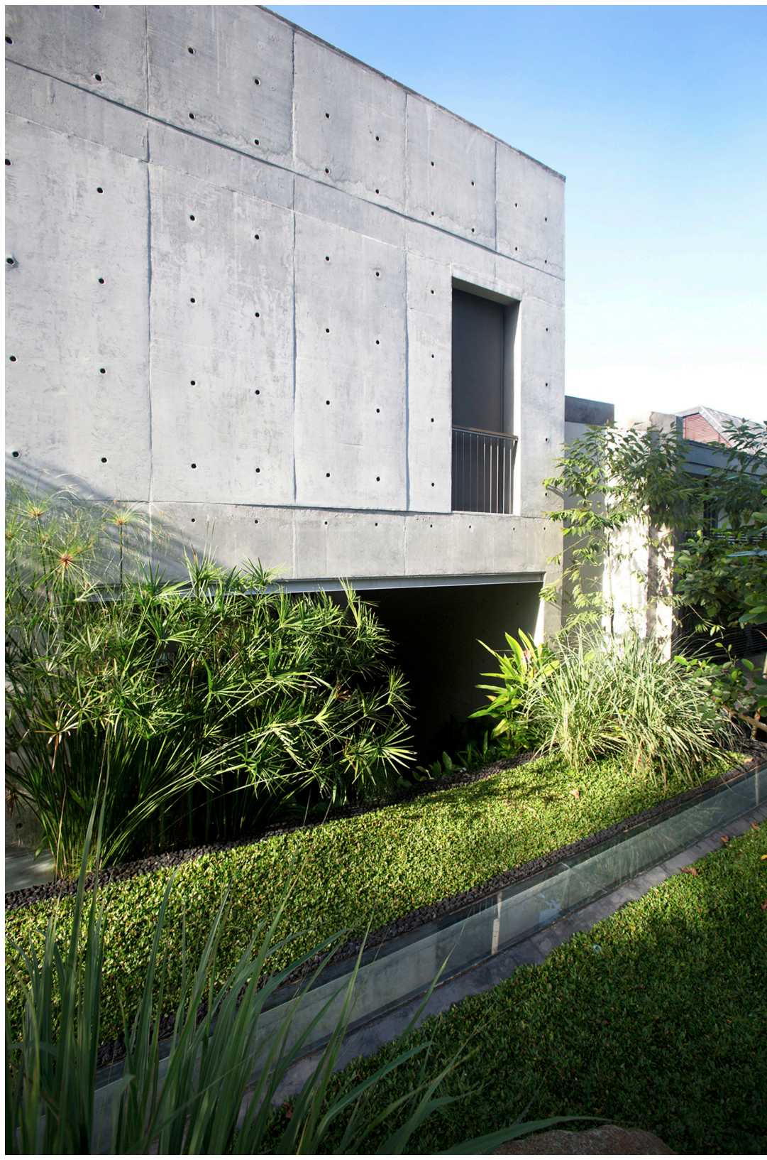
II. 4.48. Channg Architects, Namly House .
