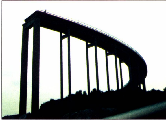
Fig. 2. The Almö Bridge after the collapse (By courtesy of Chalmers University of Technology Göteborg)
