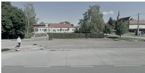
Fig. 6. Google Streetview about Dány village at the examined area. Source: https://maps.app.goo.gl/vjxsjBDtAzjmqS7DA (date of access: 2022)
